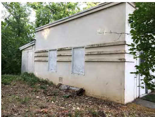
Figure 82: Western elevation of ROP Classroom (Utility Building/Garage) with boarded-up windows and exterior shed at left. Photograph taken 6/24/2019.
