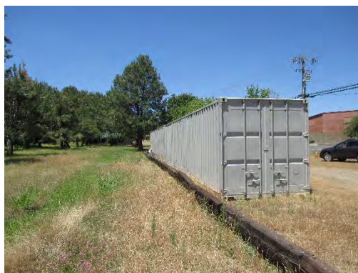
Figure 297: Southern and eastern elevations, with retaining wall over remains of Stone Run. Photograph taken 6/26/2019.
