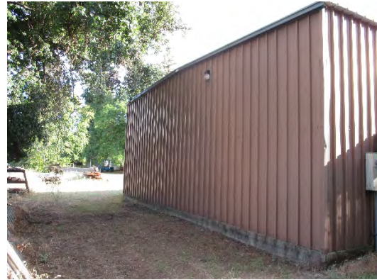
Figure 251: Eastern elevation of Shop/Storage Building (Old Search-and-Rescue) with no windows, doors, or other architectural features. Photograph taken 6/25/2019.
