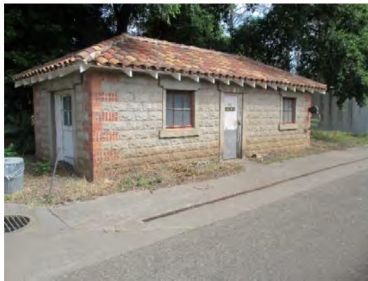
Figure 95: View of Tankhouse (Pumphouse) from the northwest. This building, constructed ca. 1905, is the only existing building on the present-day site of the Chico Plant Introduction Garden that does not markedly display a post Arts-and-Crafts movement modern style of American architecture. Photograph taken 6/25/2019.
