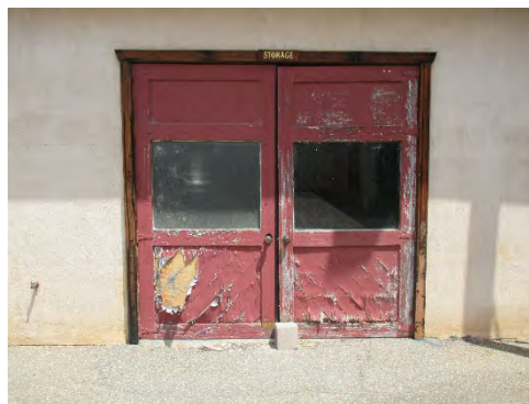
Figure 121: One of four double-doors on interior courtyard of headhouse. Photograph taken 6/25/2019.
