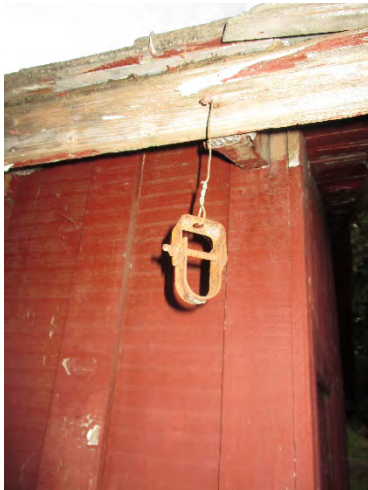
Figure 236: Hardware fixture hanging from wire at the southeastern corner of building. Photograph taken 6/25/2019.
