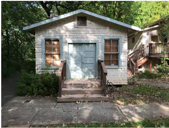
Figure 64: Western elevation and primary entrance of Office Annex Building. Office Building (Laboratory) on the right. Photograph taken 6/24/2019.
