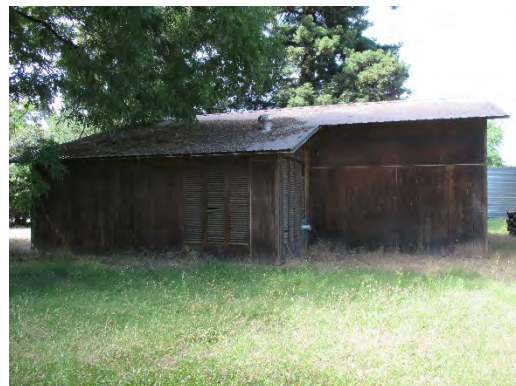
Figure 178: Southern elevation of Tree Cooler 3 of 3 (Willamette Barn). Photograph taken 6/25/2019.
