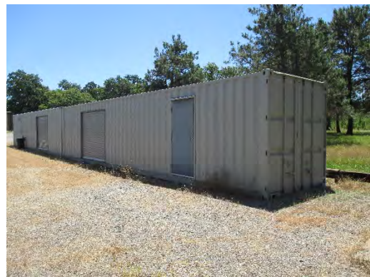
Figure 296: Northern and western elevations. Photograph taken 6/26/2019.
