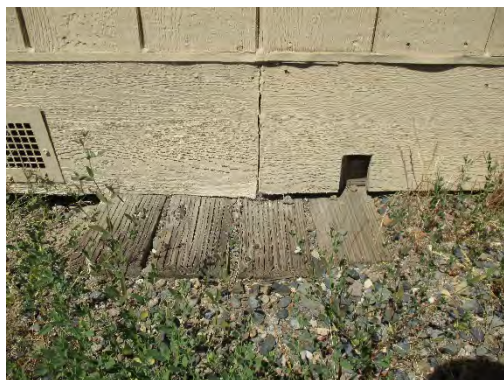
Figure 293: Horizontal baseboards and foundation of wooden boards. Photograph taken 6/26/2019.
