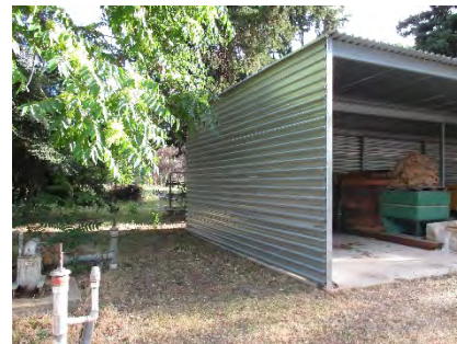
Figure 267: Eastern elevation of structure. Note historic east well at left. Photograph taken 6/25/2019.
