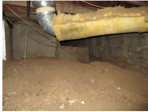
Figure 51: Original concrete front steps up to the pre-1941 front porch of the southern elevation. These steps are now enclosed by the concrete perimeter foundation of the 1941 southern addition. Photograph taken 6/24/2019.
