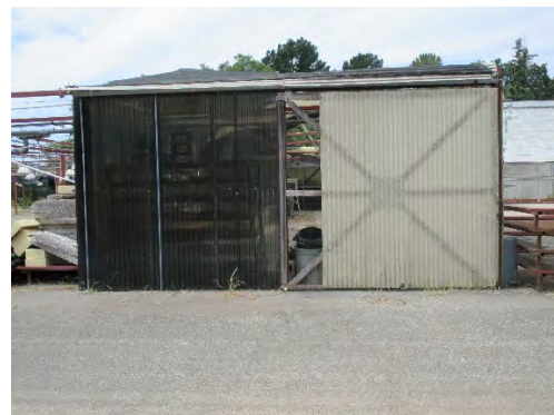
Figure 151: Wood-framed sliding door to 'room' at northeast portion of structure, just south of greenhouse (on right). Photograph taken 6/25/2019.
