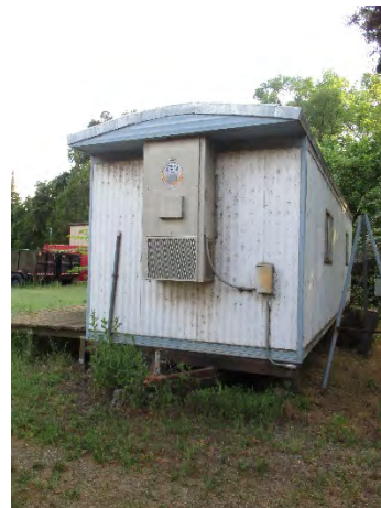
Figure 263: Eastern elevation of mobile office, with roof overhang overtop affixed air-conditioning unit and other utilities. Two double-paned casement windows of northern elevation are visible on the right, and the Storage Building (Warehouse) is visible at back left. Photograph taken 6/25/2019.
