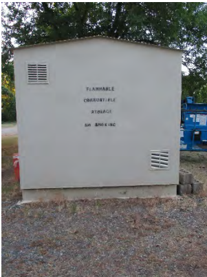
Figure 272: Southeastern façade of flammables and combustibles storage container, with two flat grate vents. Photograph taken 6/25/2019.
