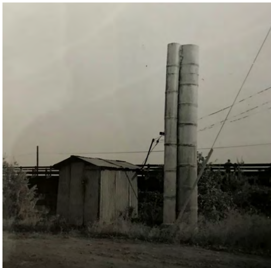
Figure 240: Butte Creek Pumphouse and adjacent irrigation standpipes. Photograph taken on November 16, 1959.
