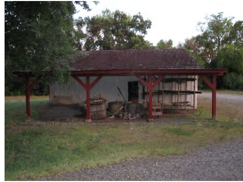
Figure 235: Northern elevation of Barn with unenclosed porch addition. Photograph taken 6/25/2019.
