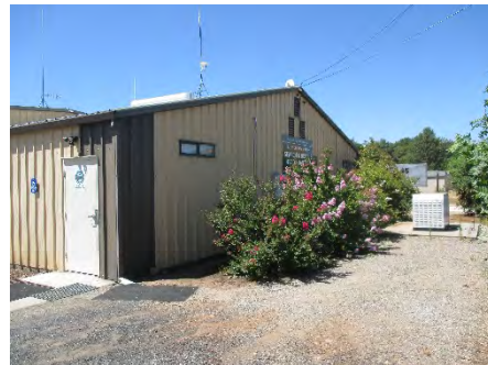
Figure 280: Northern façade of Butte County Sheriff Search and Rescue Headquarters, with flowering shrubs obscuring utilities. Photograph taken 6/26/2019.
