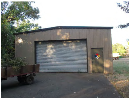
Figure 268: Southwestern primary elevation of Storage Building (Warehouse), with pedestrian entrance and vehicle bay door fronting on asphalt driveway. Photograph taken 6/25/2019.
