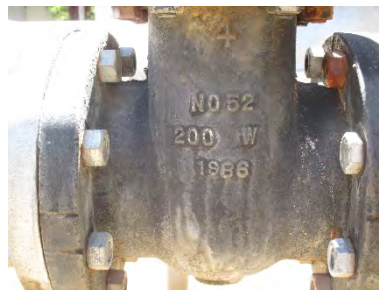
Figure 310: Steel joint of the south well, embossed with “4; NO 52; 200 W; 1986.” Photograph taken 6/26/2019.
