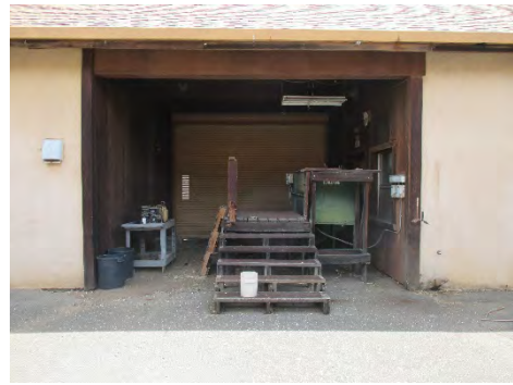
Figure 135: One of three breezeways, as seen from interior of courtyard. Photograph taken 6/25/2019.
