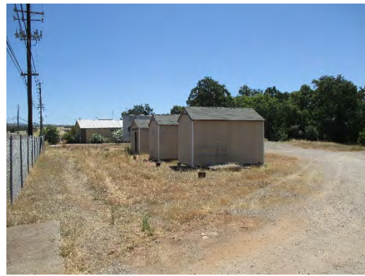
Figure 300: Three of five new search-and-rescue storage sheds with Search and Rescue Headquarters in background. Photograph taken 6/26/2019.
