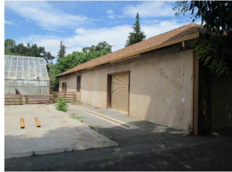
Figure 131: Southern elevation of headhouse. Greenhouse to the left. Photograph taken 6/25/2019.
