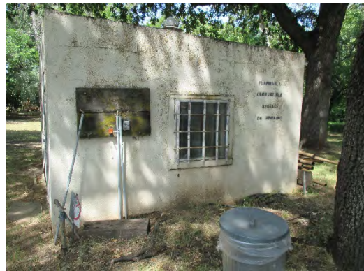
Figure 116: Eastern elevation of Saw/Paint Storage Building (Fumigation Storage), with the building's only window. Photograph taken 6/25/2019.
