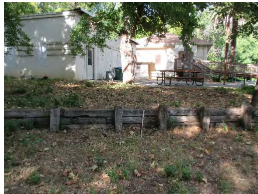
Figure 87: Retaining wall of railroad-tie cribbing. Utility building on left. Office Building (Laboratory) in background. Photograph taken 6/24/2019.
