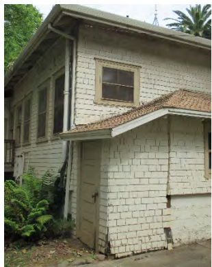
Figure 38: Early one-room addition at northwestern corner of building. Photograph taken 6/24/2019.
