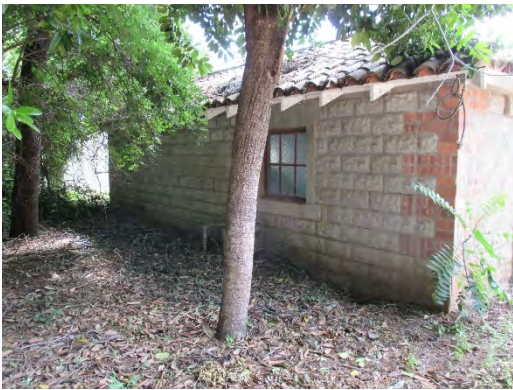
Figure 102: Eastern elevation of Tankhouse (Pumphouse) with exotic plantings in foreground. Photograph taken 6/25/2019.
