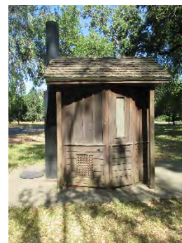
Figure 325: Eastern façade. Photograph taken 6/26/2019.
