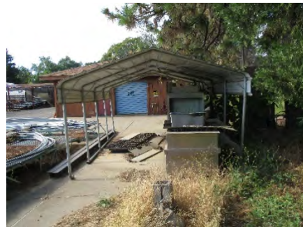
Figure 188: Shade canopy with Pump/Injector Building in the background. Photograph taken 6/25/2019.
