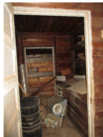
Figure 239: Small front 'office' area of the Barn. Photograph taken 6/25/2019.
