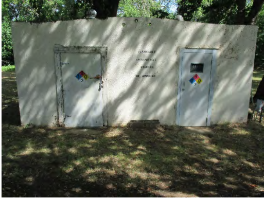
Figure 113: Southern (primary) elevation of Saw/Paint Storage Building (Fumigation Storage) with decorative three-hole motif at center of roofline. Photograph taken 6/25/2019.
