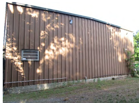
Figure 253: Western elevation of Shop/Storage Building (Old Search-and-Rescue) with one awning-style window of three single horizontal panes. Photograph taken 6/26/2019.
