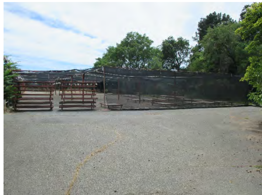
Figure 158: Northern elevation of shadehouse. Photograph taken 6/25/2019.
