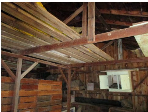
Figure 238: View of interior wood framing of the Barn. Photograph taken 6/26/2019.
