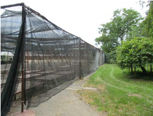
Figure 157: Western elevation of shadehouse, with father kiwi at right. Photograph taken 6/25/2019.
