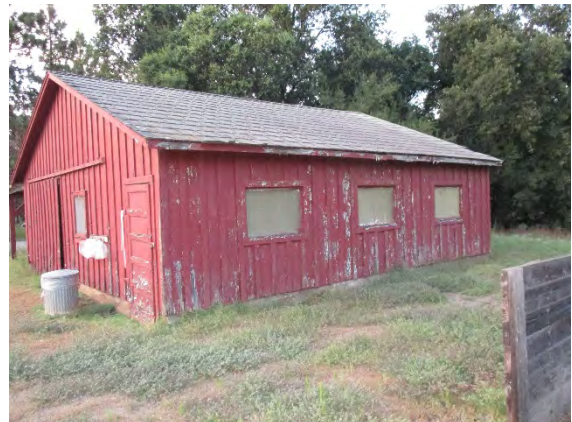
Figure 233: Southern elevation of Barn, with three windows that have been fitted with plastic. Photograph taken 6/25/2019.
