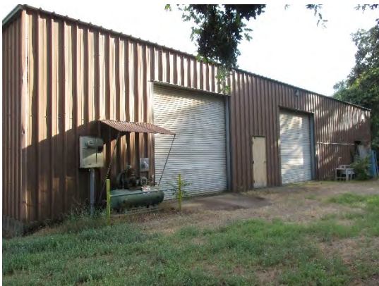
Figure 252: Northern (riverside) elevation of Shop/Storage Building (Old Search-and-Rescue), with pedestrian entrance, two roll-up vehicle bay doors, and two canopy awnings overtopping utilities. Photograph taken 6/26/2019.
