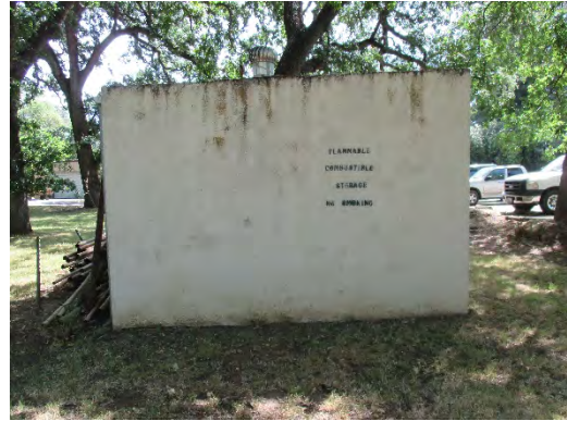
Figure 114: Western elevation of Saw/Paint Storage Building (Fumigation Storage). Photograph taken 6/25/2019.
