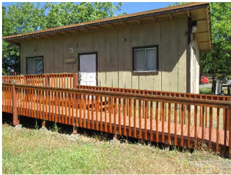
Figure 283: Primary southern elevation of O.C. Crew Office Building, with open front deck and ramp. Photograph taken 6/26/2019.
