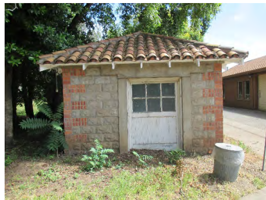
Figure 103: Northern elevation of Tankhouse (Pumphouse) with secondary sliding-door entrance. Photograph taken 6/25/2019.
