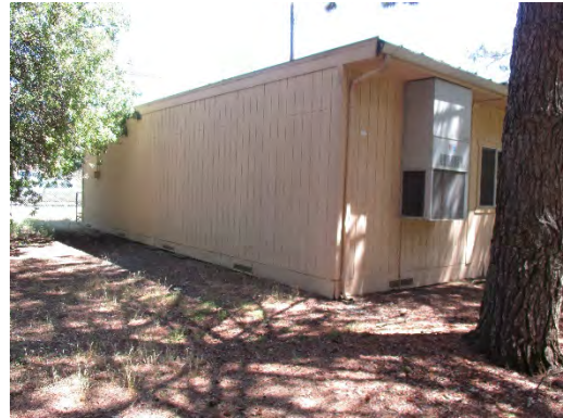
Figure 292: Western elevation with no windows or doors. Photograph taken 6/26/2019.
