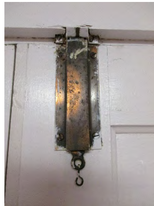
Figure 61: One example of original hardware of front door of Office Annex Building. Photograph taken 6/24/2019.
