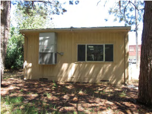
Figure 291: Southern elevation with one casement window and affixed air-conditioning unit. Photograph taken 6/26/2019.
