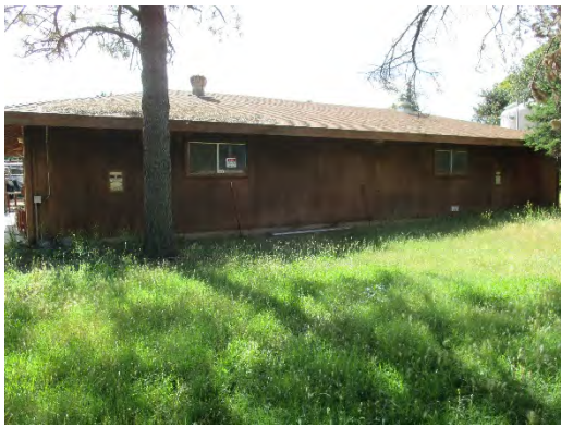
Figure 167: Eastern elevation of Pump/Injector Building. Photograph taken 6/25/2019.
