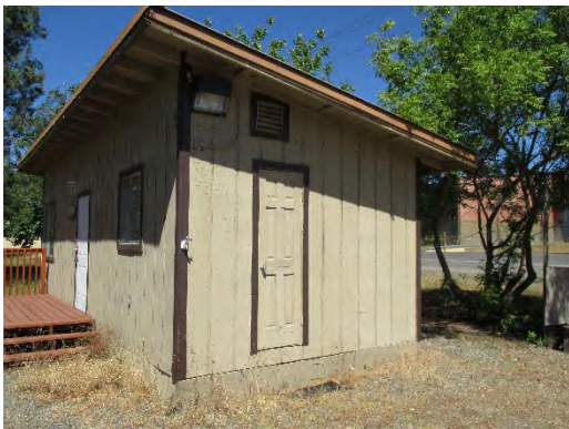
Figure 285: Eastern elevation with door raised above ground level. Photograph taken 6/26/2019.
