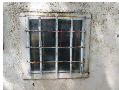
Figure 109: The only window of the Saw/Paint Storage Building (Fumigation Storage), on its eastern elevation. Photograph taken 6/25/2019.
