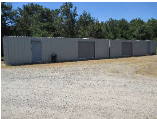
Figure 295: Northern (roadside) elevation of two fire cache containers, located within the Search and Rescue Headquarters building cluster. Photograph taken 6/26/2019.
