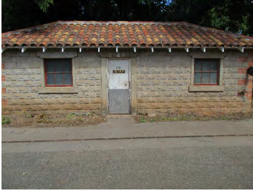
Figure 100: Western elevation of Tankhouse (Pumphouse), with primary entrance. Photograph taken 6/25/2019.
