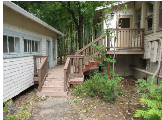
Figure 47: Wooden back porch, north of building, connecting Office Building (Laboratory) on right to Office Annex Building on left. Photograph taken 6/24/2019.
