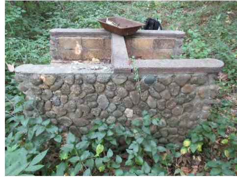
Figure 91: Side view of two-sided grill, showing mortared river-cobble construction. Photograph taken 6/24/2019.
