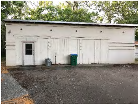
Figure 80: Southern (roadside) elevation of the ROP Classroom (Utility Building/Garage). Photograph taken 6/24/2019.
