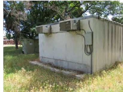
Figure 182: Eastern elevation of cold-storage shed, with two air-conditioning units at roof-wall junction. Photograph taken 6/25/2019.
