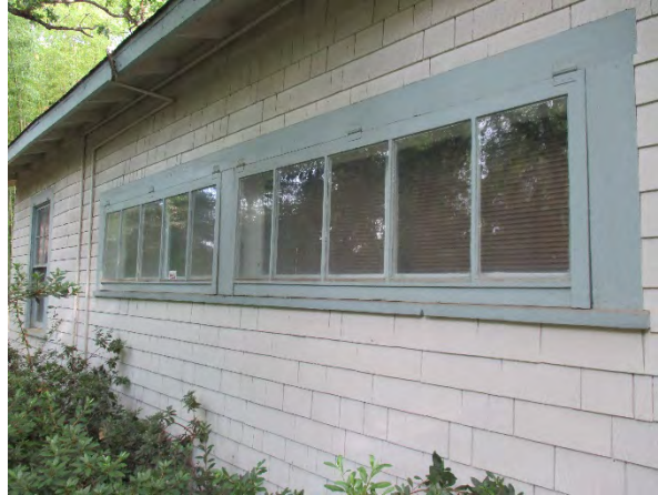
Figure 59: Window ribbons characteristic of the ranch style of domestic architecture, located on the northern elevation of the Office Annex Building. Photograph taken 6/24/2019.
