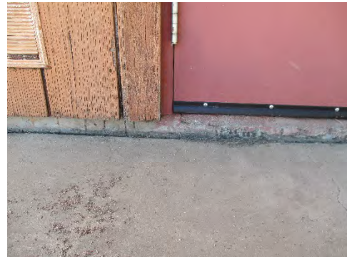
Figure 170: Concrete slab foundation. Photograph taken 6/25/2019.
