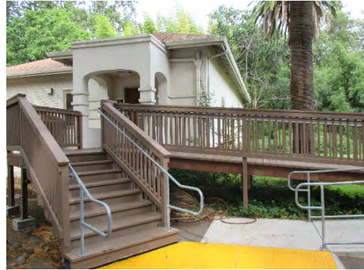
Figure 45: Accessible wooden ramp, built after 1991, leading to the main entrance at southwestern corner of building. Photograph taken 6/24/2019.
