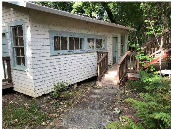
Figure 65: Southern elevation of Office Annex Building with back deck. Photograph taken 6/24/2019.
