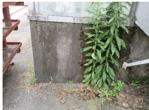
Figure 149: 1-2' poured concrete perimeter foundation. Photograph taken 6/25/2019.
