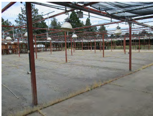
Figure 159: Interior of shadehouse with light fixtures and irrigation sprinklers hanging from overhead steel beams . Photograph taken 6/25/2019.
