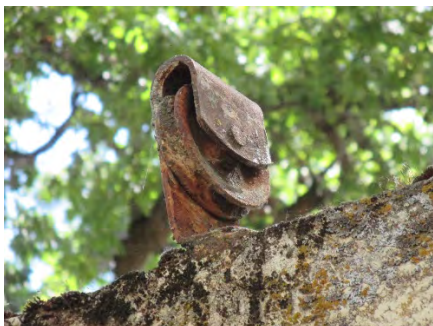
Figure 110: Old pulley system at roof-wall junction of western elevation. Photograph taken 6/25/2019.
