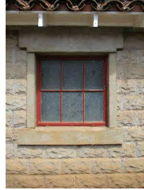
Figure 97: Window from western elevation of Tankhouse (Pumphouse). Note thick concrete pediment. Photograph taken 6/25/2019.
