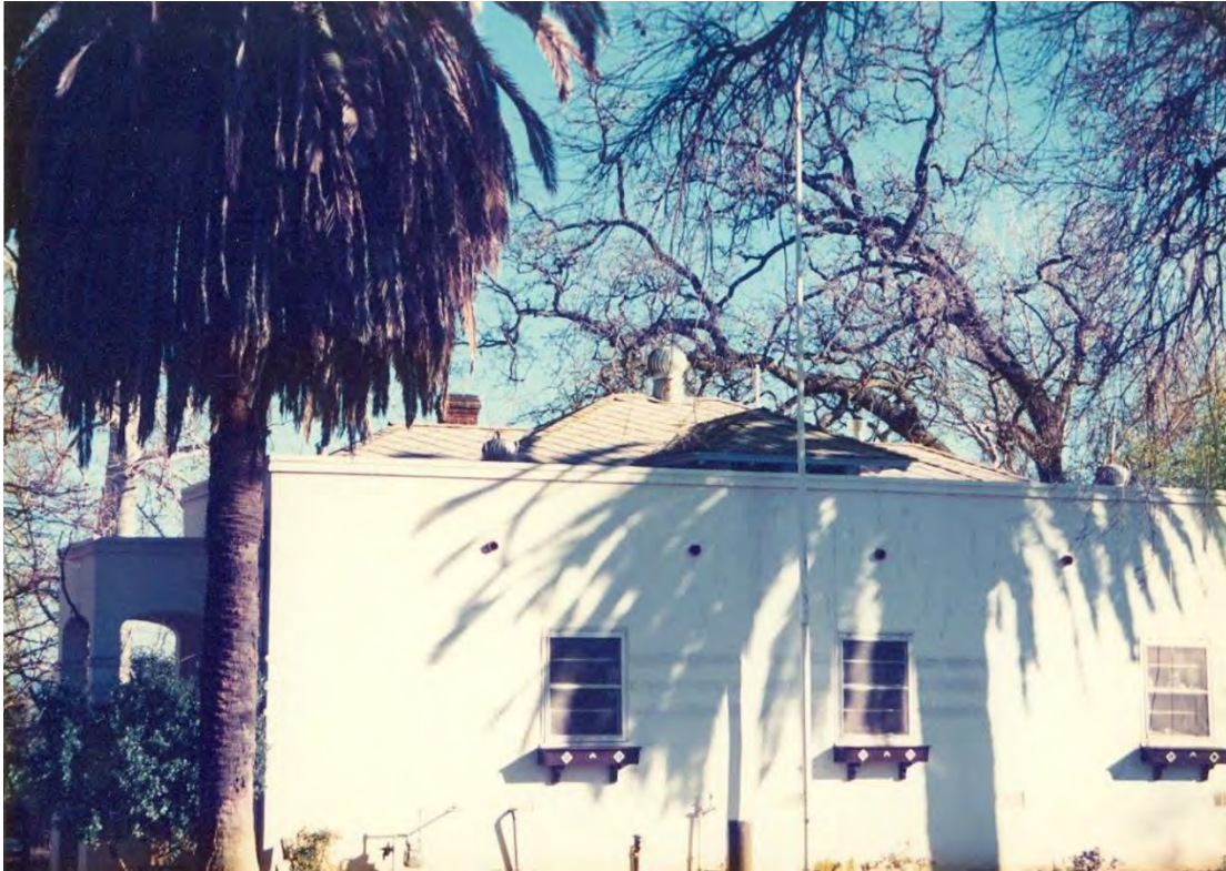
Figure 30: The southern façade of the Office Building (Laboratory) and arched entryway to left. Note coping at the roof line and discoloration left by three embossed horizontal bands (since removed at time of photograph). Also note hipped dormer from original roof, visible above flat roof of addition. Photograph taken March 1, 1990.
