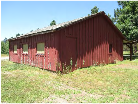
Figure 234: Eastern elevation of Barn with one solid metal door and one boarded-up window. Photograph taken 6/26/2019.
