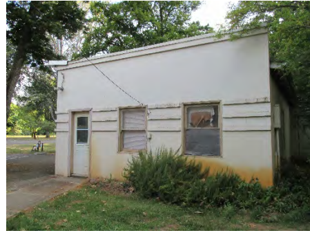
Figure 81: Eastern elevation of the ROP Classroom (Utility Building/Garage), originally the primary pedestrian access. The center window is the only window left on the building with both intact sashes. Photograph taken 6/24/2019.
