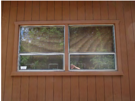
Figure 122: Paired windows on western elevation in post-1950 metal frames. Photograph taken 6/25/2019.
