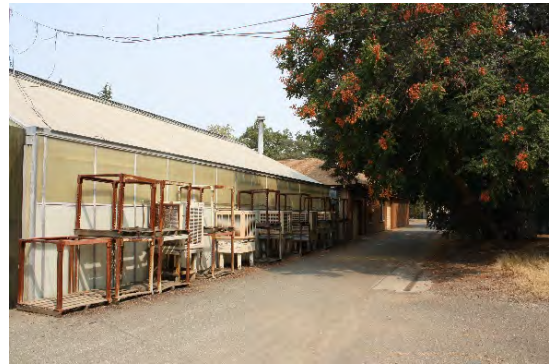
Figure 25: Eastern façade of fiberglass-and-aluminum greenhouse removed from site in late 2018. Photograph taken 8/20/2015. Photograph courtesy of Joel Little.
