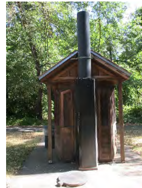
Figure 323: Southern façade with large ventilator. Photograph taken 6/25/2019.
