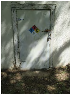
Figure 106: Left-hand door of southern (primary) elevation. Photograph taken 6/25/2019.
