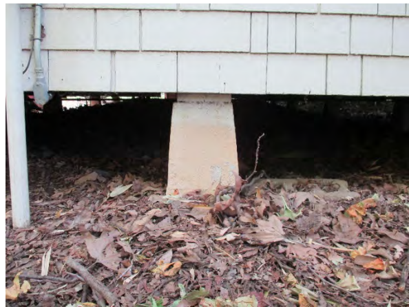
Figure 57: Thick wooden shim atop foundation of concrete pier block. Photograph taken 6/24/2019.
