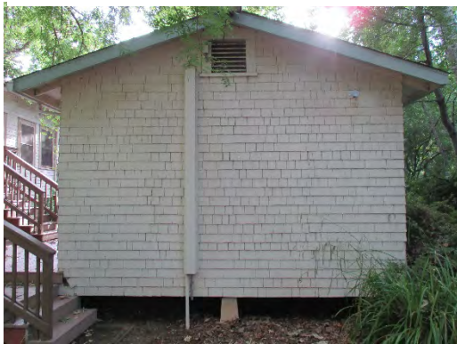
Figure 66: Eastern elevation of Office Annex Building. Photograph taken 6/24/2019.
