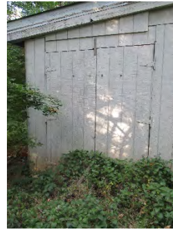
Figure 85: Western double-door entrance to exterior shed. Photograph taken 6/24/2019.
