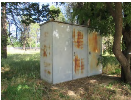
Figure 183: Western elevation of smaller southern cold-storage shed. Photograph taken 6/25/2019.
