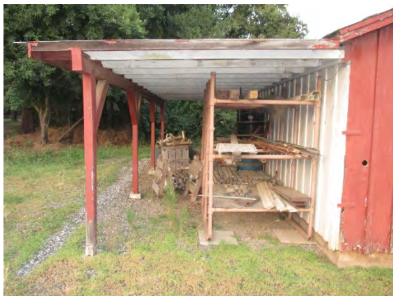
Figure 230: Post-1979 porch addition. Photograph taken 6/25/2019.
