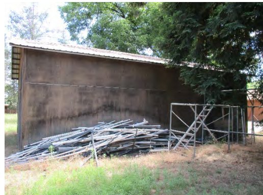
Figure 180: Northern elevation of Tree Cooler 3 of 3 (Willamette Barn). Photograph taken 6/25/2019.
