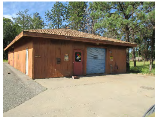
Figure 166: Southern elevation of Pump/Injector Building, with vehicle drive-up bay and grove of mostly exotic trees in background. Photograph taken 6/25/2019.
