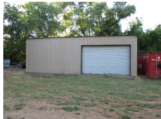
Figure 269: Southeastern elevation of warehouse/storage building with vehicle bay door fronting on the Shop Road maintenance yard. Adjacent 'K-Line' container is located directly northeast of the building. Photograph taken 6/25/2019.
