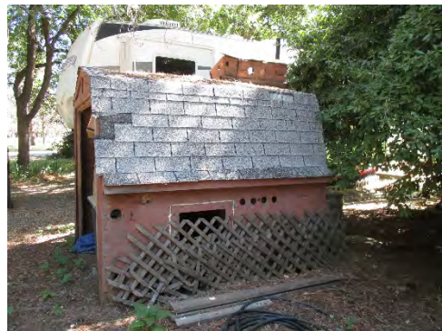
Figure 317: Southern façade of storage shed, showing gambrel roof with bottom flange. Note modifications presumably for use as a doghouse. Photograph taken 6/26/2019.
