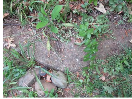
Figure 77: Aggregate concrete slab foundation with pebble inclusions. Photograph taken 6/24/2019.
