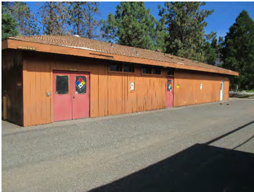
Figure 165: Western (primary) elevation of Pump/Injector Building. Photograph taken 6/25/2019.
