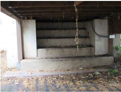
Figure 52: 1941 concrete steps leading to art moderne arched entryway. These steps are now obscured beneath the wooden accessible ramp, installed after 1991. Photograph taken 6/24/2019.
