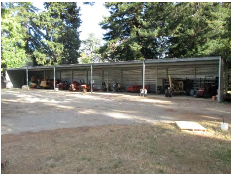
Figure 264: Open northern elevation of Open Garage. Photograph taken 6/25/2019.
