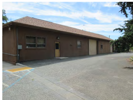
Figure 129: Western elevation of headhouse. Photograph taken 6/25/2019.
