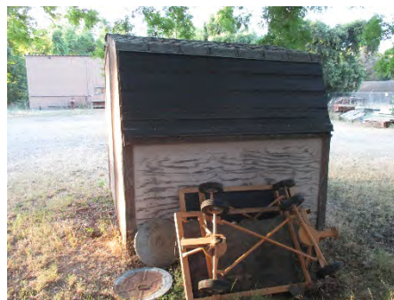
Figure 259: Southeastern façade of Shop Road small storage shed, with Shop/Storage Building (Old Search-and-Rescue) in the background. Photograph taken 6/25/2019.
