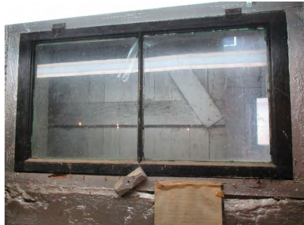
Figure 34: Basement-level window with carved wooden window-stop. Photograph taken 6/24/2019.
