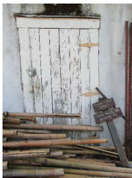
Figure 108: Unused wooden shed door on northern elevation. Photograph taken 6/25/2019.
