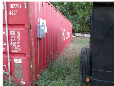
Figure 275: Eastern façade of Shop Road K-line container with utility hook-up for electric floodlight fixture. Photograph taken 6/25/2019.
