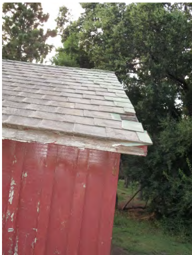
Figure 226: Horizontally overlapping roof shingles. Photograph taken 6/25/2019.
