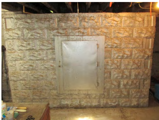
Figure 35: Basement storage room, patented 1870, constructed ca. 1907. Photograph taken 6/24/2019.
