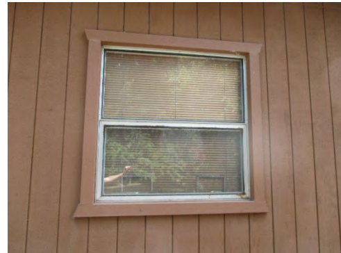
Figure 123: Non-paired window variation on western elevation. Photograph taken 6/25/2019.
