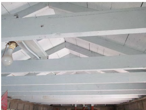
Figure 104: Exposed boards and rafters on interior of Tankhouse (Pumphouse). Photograph taken 6/25/2019.
