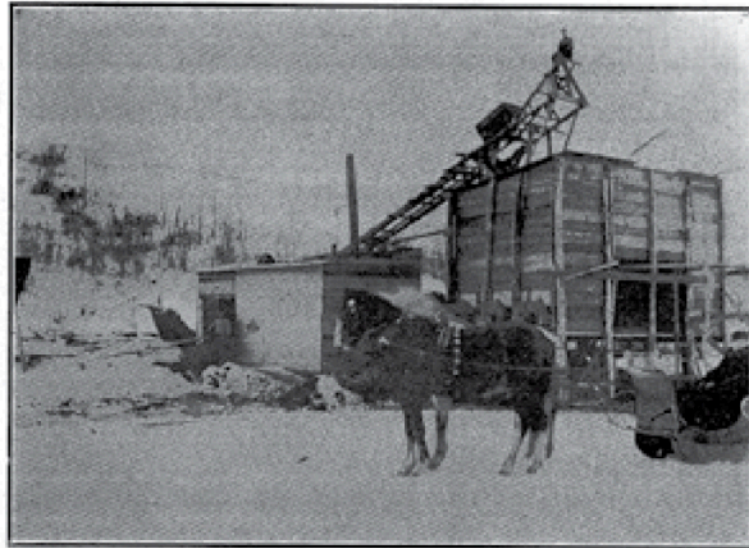
A Primitive Coal Mine in the Camrose District. Many farmers have private mines and supply coal to their immediate neighborhood at from $2 to $3 per ton.
