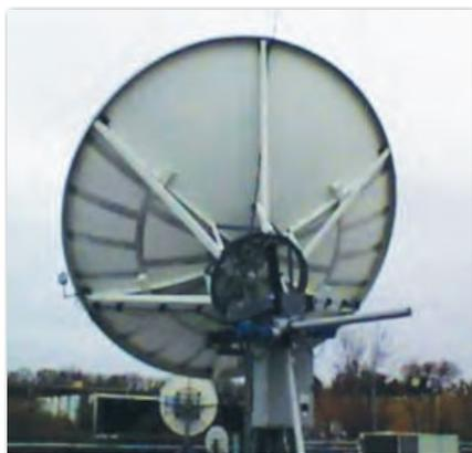
Figure 1: Antenna Rear – Surface / Pad Heated Anti-icing
