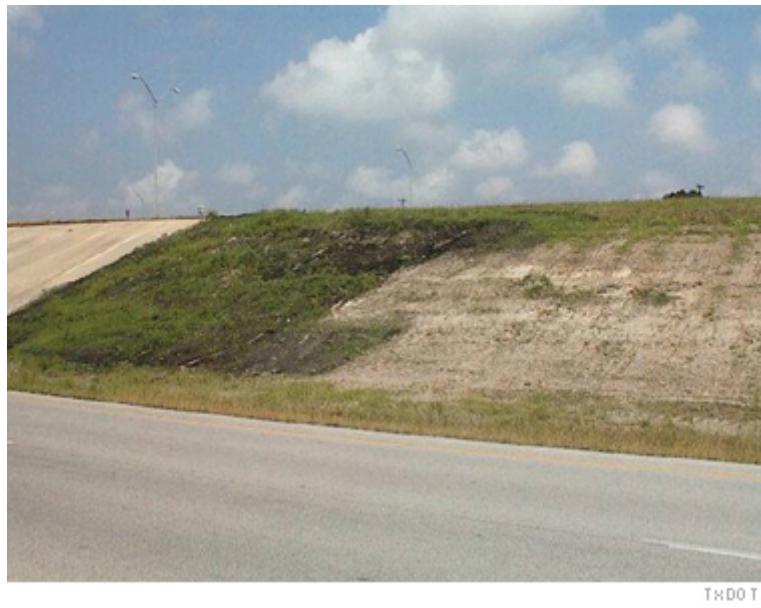
(After) TxDOT smoothed the slope and applied erosion control compost. This photo shows the same slope 2 weeks after compost was applied.
