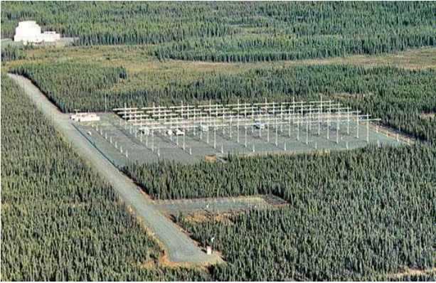
Fig. 3 The main element of the HAARP project 27 : a powerful array of 180 radio emitters, capable of generating 3,6MW of electromagnetic power in the 2-10MHz frequency range (2010). Alaska, USA. Coordinates = (63°32'30"N, 145°09'03"W).
