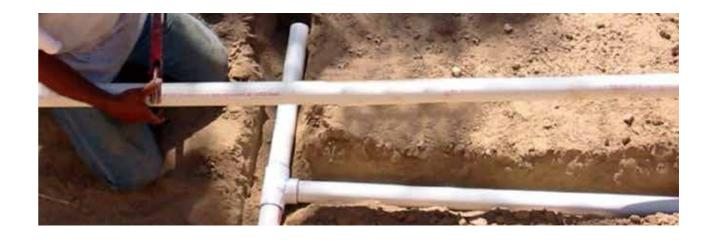
1. The trench should be excavated to ensure the sides will be stable under all working conditions. The trench should be
