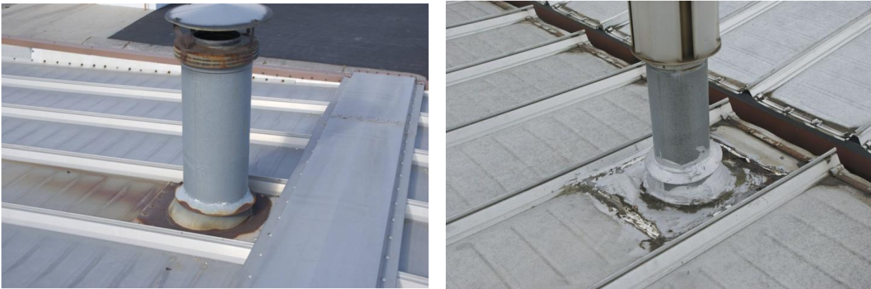
Figure 19 – Two examples of flashing round penetrations.
