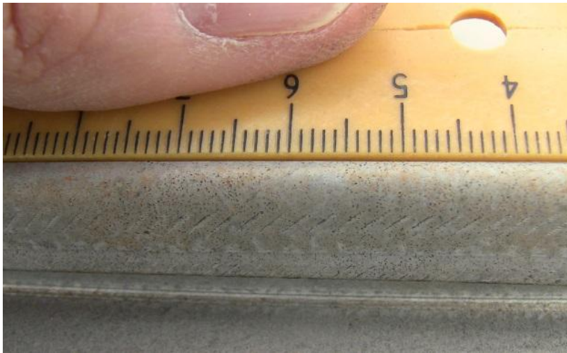
Figure 12 – Excellent performance (only brownish dirt pick-up) along the top radius of a standing seam on a 29-year old roof in Athens, GA.
