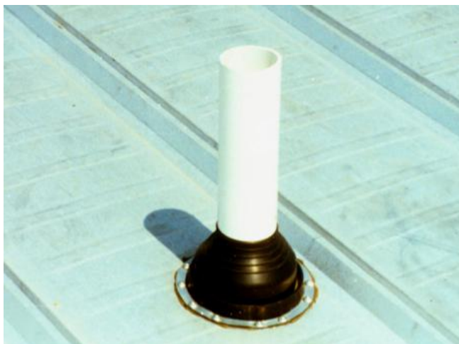
Figure 2 – Best-practice flashing of round roof penetration.
