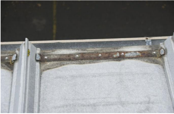
(c) 300 series SS cap screws at 31 years
