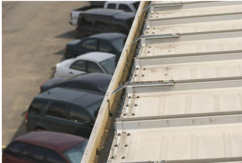
Figure 22 – Typical gutter manufactured from prepainted galvanized G-90 steel.
