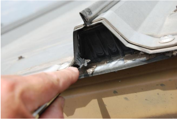
Figure 16 – Typical eave closure.
