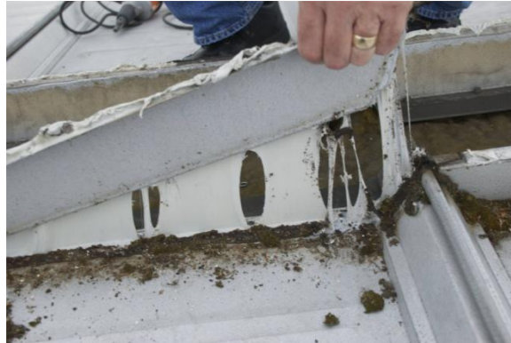
Figure 17 – Typical ridge closure.
