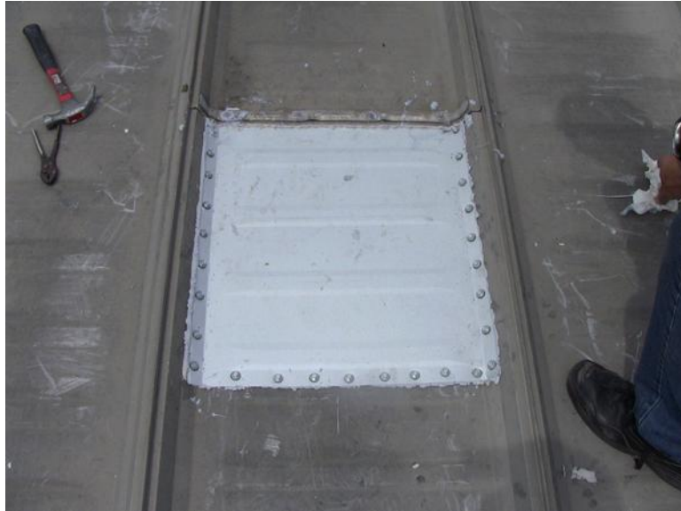
Figure 9 – Completed patch after removal of exposed sample.
