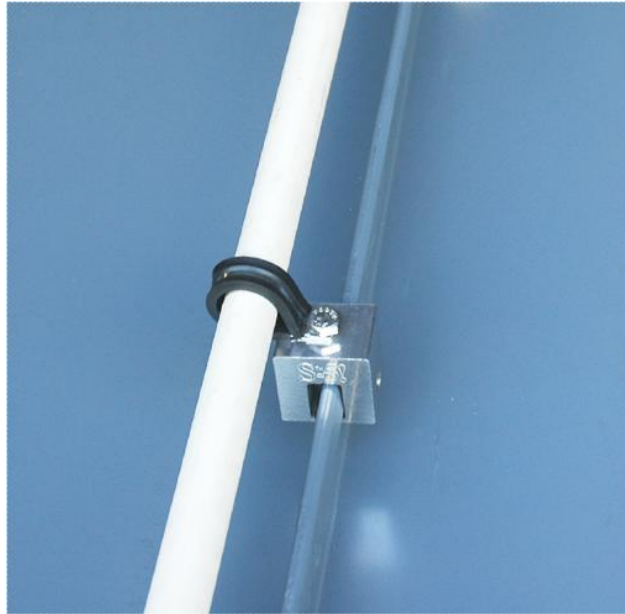
Figure 3 – Best practice is to carry condensate to the eave or a vent pipe using PVC piping properly mounted to the roof panels to avoid premature corrosion of the 55% Al-Zn alloy coating of roof panels.
