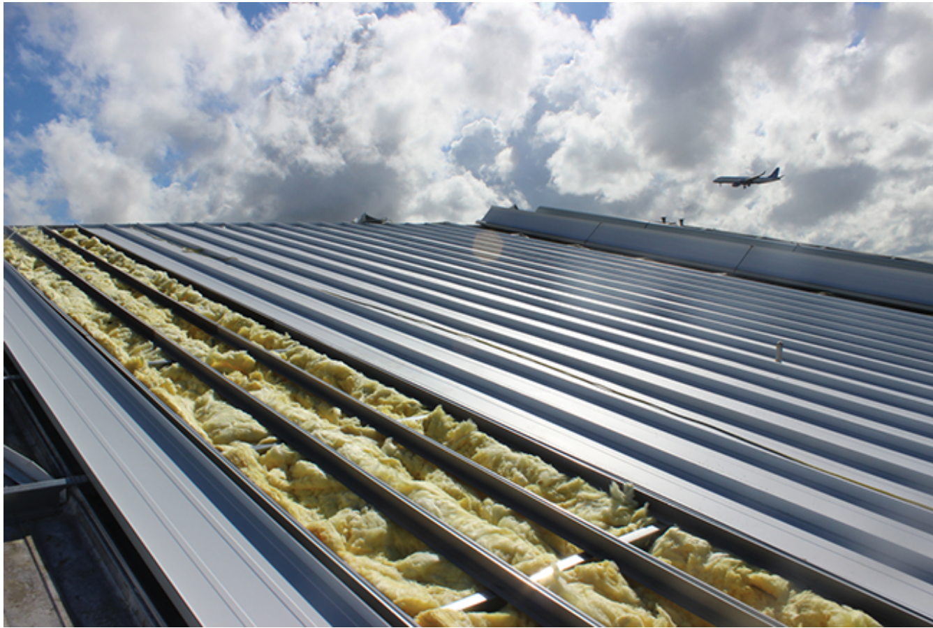
Figure 2: Metal roof installation in progress over an existing metal roof
