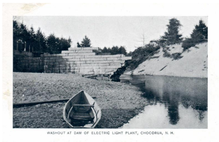
Postcard of the flood damage to the dam in 1916
