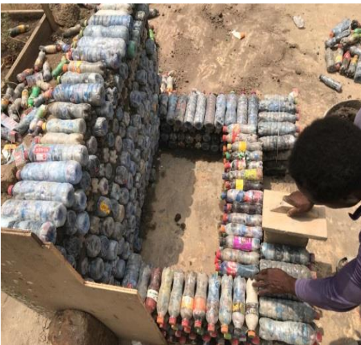
Start forming the throne with MORE ecobricks
