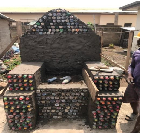
Fill the sit of throne with sand and cement throne
