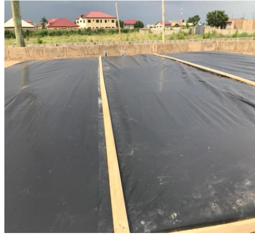
Cover the top of the insulation box with 6mill black plastic shown
