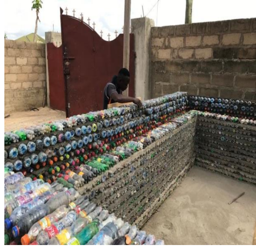
Raising the outside walls as shown.
