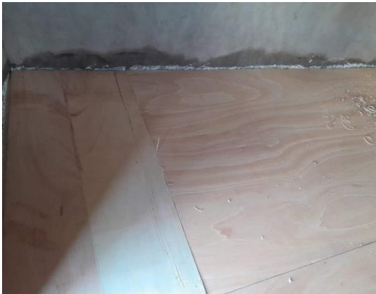
Insulating inside floor with EPS foam and plywood as shown
