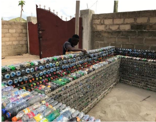
Carefully arrange the ecobricks
