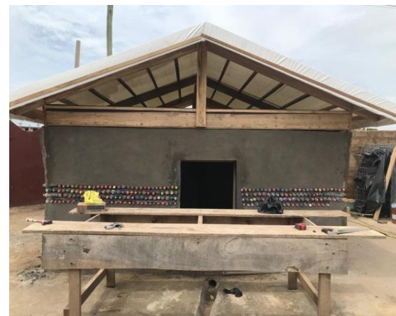
Frame the roof and cover with white Tarp as shown
