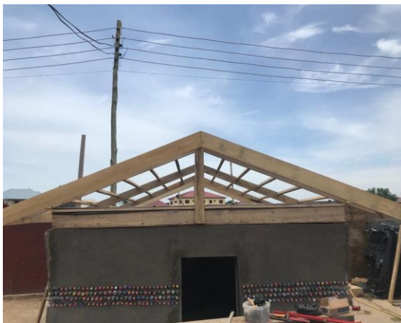
Frame the roof and cover with white Tarp as shown
