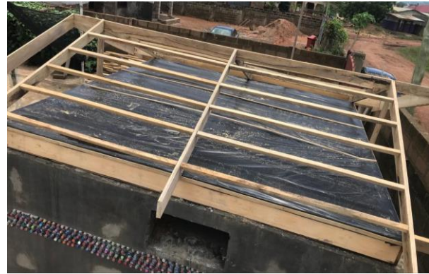
Errect a ridge beam and wood trusses on top of the cold storage space
