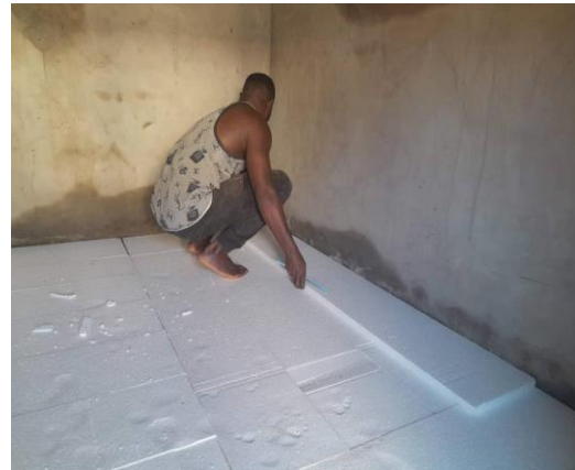
Insulating inside floor with EPS foam and plywood as shown
