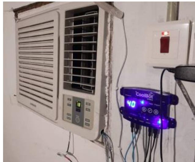
Patented temperature controller fixed inside the CSS with a compatible AC
