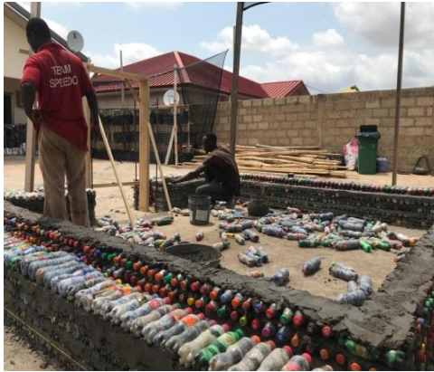
Laying of both walls as shown
