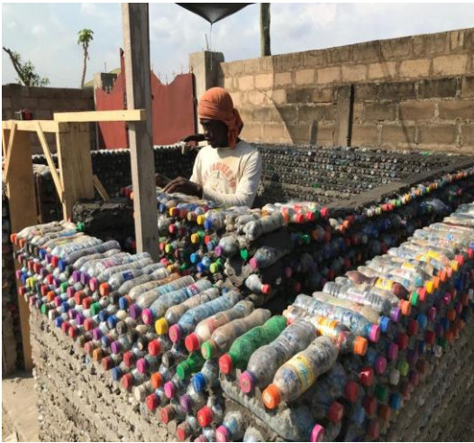
Attaching the door frame to the ecobricks
