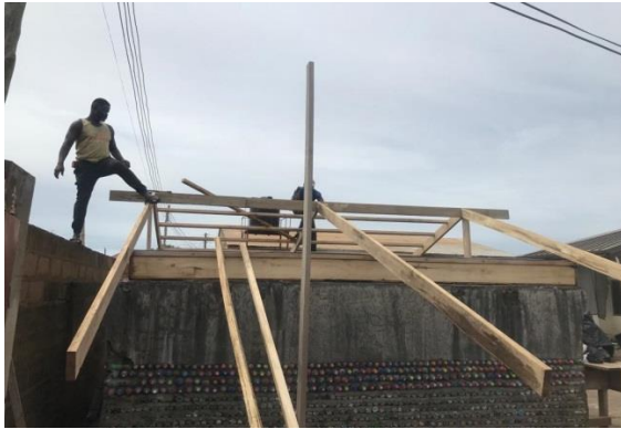
Errect a ridge beam and wood trusses on top of the cold storage space
