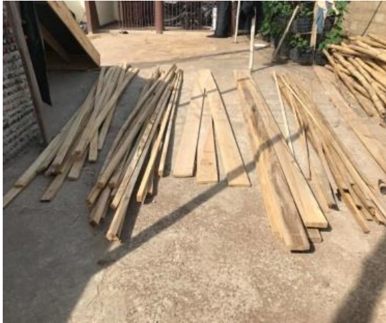
Woods for the cold storage roofing
