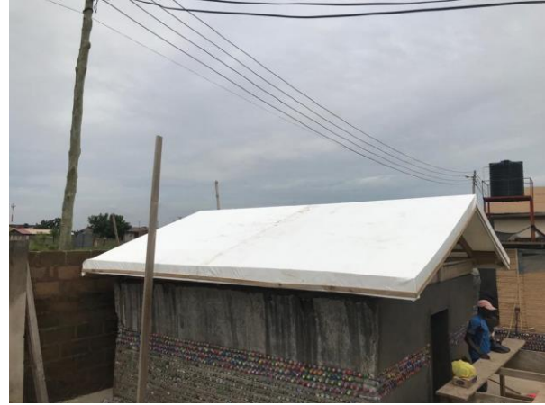
Cold storage space ready for painting
