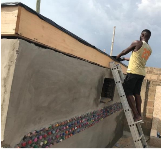
Cover the top of the insulation box with 6mill black plastic shown
