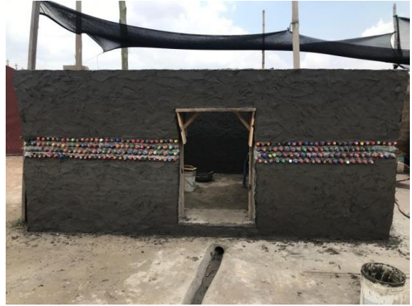
Plaster the entire walls with cement
