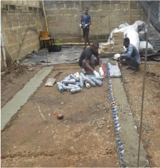
Fill the foundation with motor as shown.
