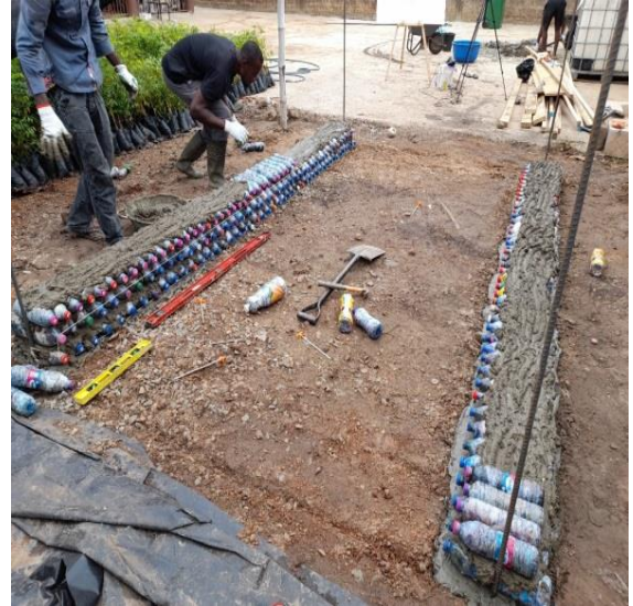
Lay ecobricks in the cement mortar.
