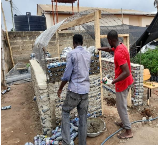
Fill in end walls with EcoBricks
