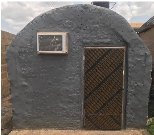
Fix the AC and door as shown
