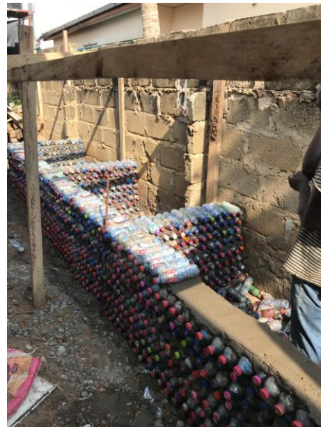
Raise EcoBricks walls to 30 inches tall as shown
