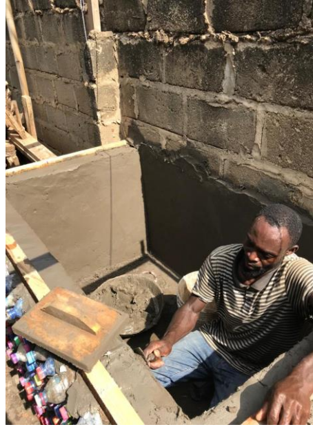
Skin coat the EcoBricks walls with cement mortar
