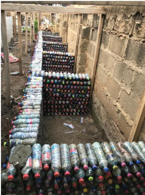
Raise EcoBricks walls to 30 inches tall as shown
