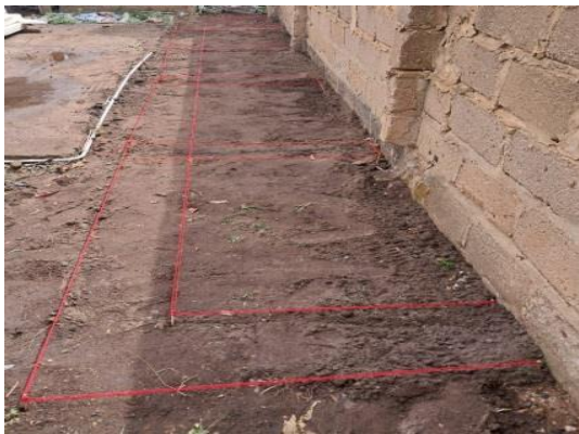
Marking the ground
