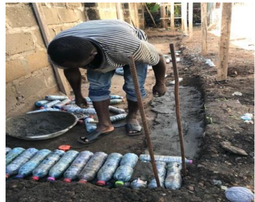
Laying the EcoBrick walls
