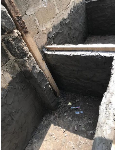
Skin coat the EcoBricks walls with cement mortar
