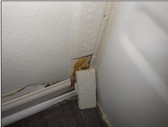
8.0 Item 1(Picture) master bathroom
