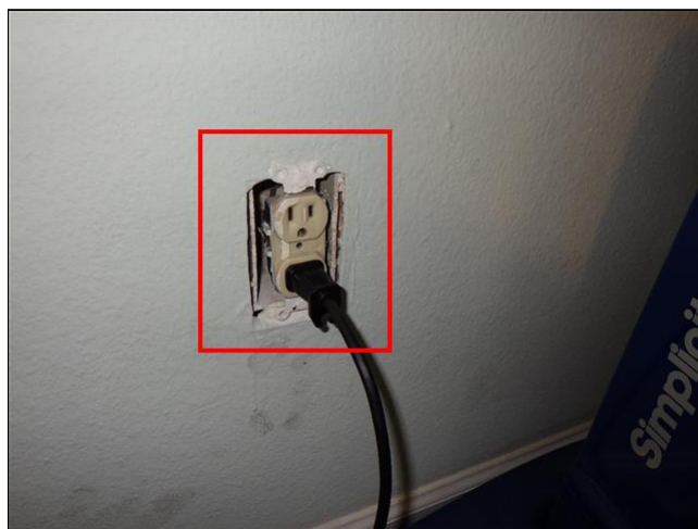
5.7 Item 4(Picture) Front right bedroom
