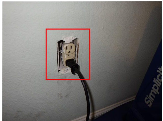
5.7 Item 4(Picture) Front right bedroom
