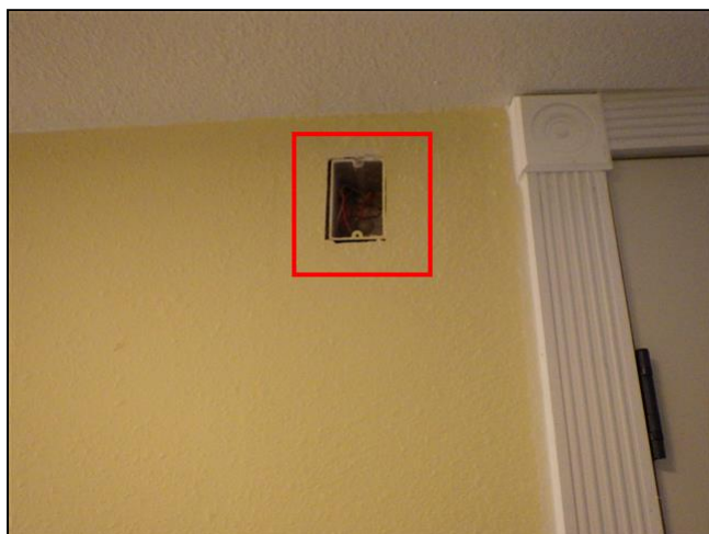
5.7 Item 3(Picture) Entry hallway
