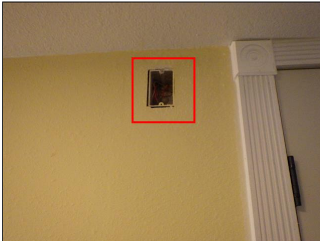
5.7 Item 3(Picture) Entry hallway
