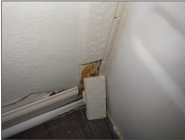
8.0 Item 1(Picture) master bathroom
