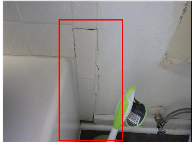
8.0 Item 2(Picture) hallway bathroom
