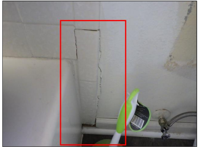
8.0 Item 2(Picture) hallway bathroom
