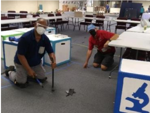
Removing studs protruding from the floor
