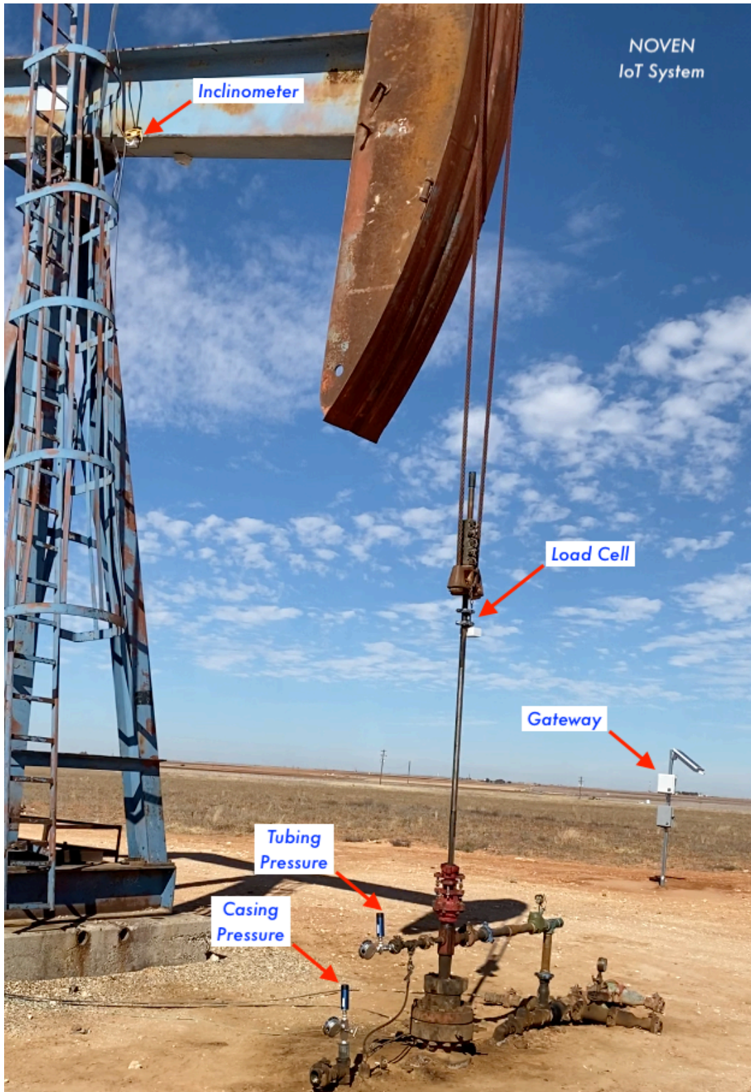
Figure 3 Typical IoT System Installation for SRP Wells
