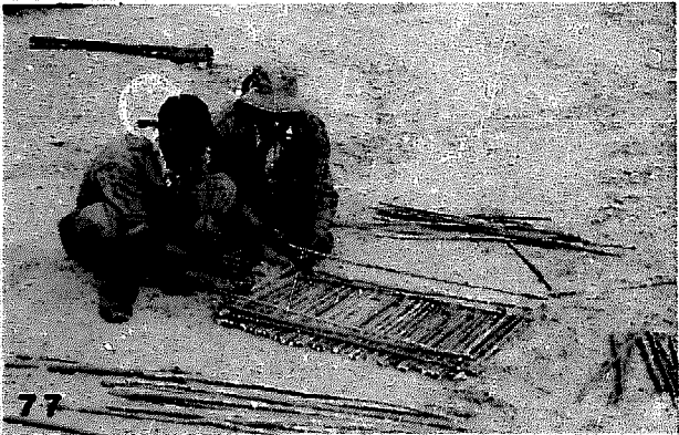
3. All sides are built up at the same time
