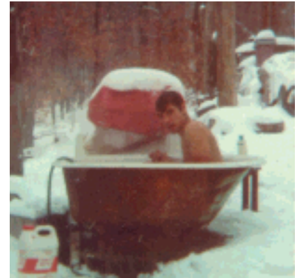
Our original plumbing system.
