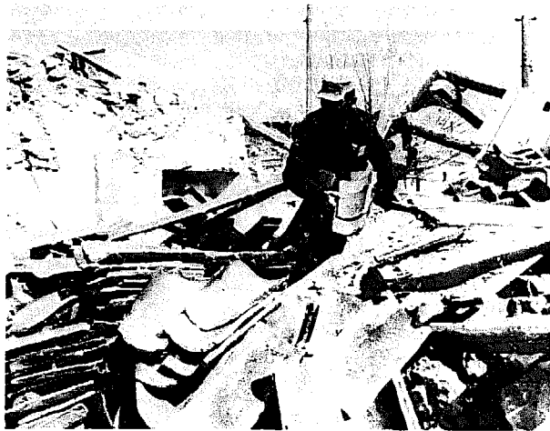
After the Corinth earthquake in Greece in March 1981, this man is salvaging roofing tiles from his damaged house.
