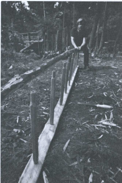
When assembling the ladder, tap the rungs in one rail, flat side up, then place the last rail on the upright rungs and align from bottom to top.
