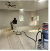
2-day process consisted of prepping the floor by grinding the surface of the concrete. This meant all the corners and edges of the floor had to be ground. The expansion cracks in the concrete were also filled. Next, a Polyurea basecoat was applied with "Autumn Harvest" flecks for texture. After drying overnight, the excess flecks were
