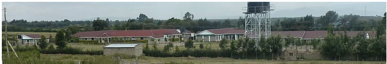
St Francis Xavier Secondary School for Girls, begun June 2006. This photo was taken November 2010.
