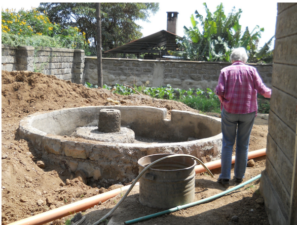
Margo inspecting the biogas installation.
