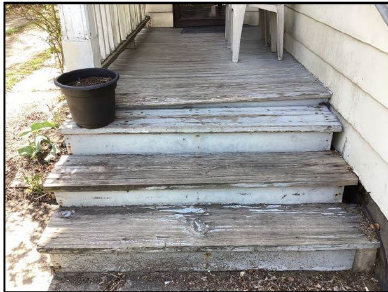
45. Seal or stain decking
