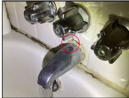
128. Second floor bathroom
