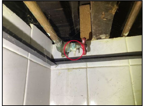
114. Corrosion
