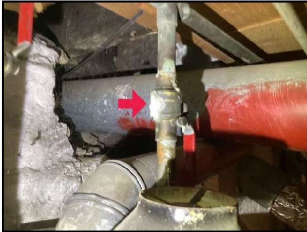
113. Corrosion
