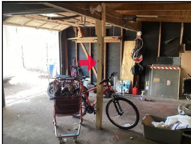
56. Additional support/s added
