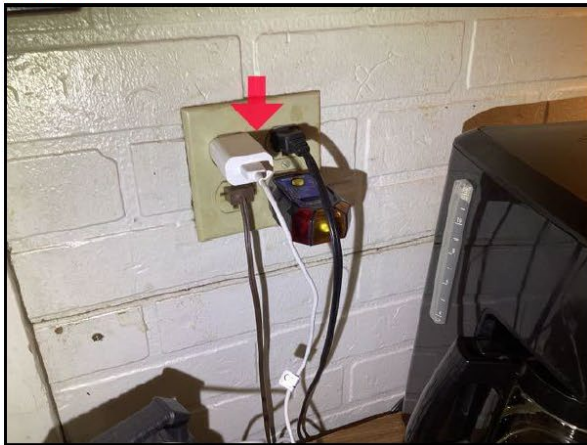
78. Ground needed for 3-slot outlet
