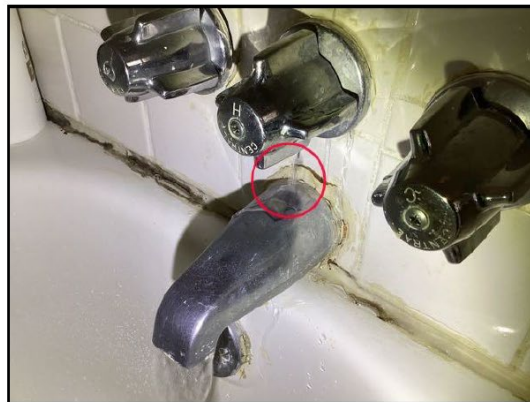
18. Second floor bathroom
