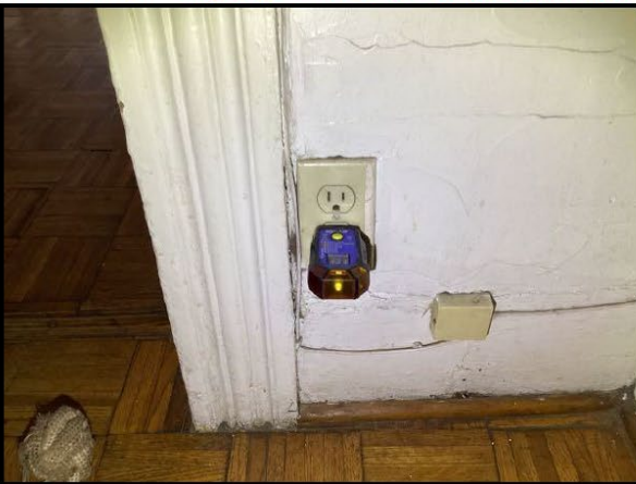
77. Ground needed for 3-slot outlet
