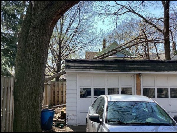
47. Trees or shrubs too close to building
