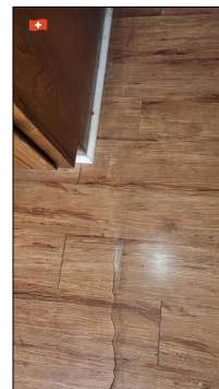
Numerous Heavy Foundation Cracks Noted.
