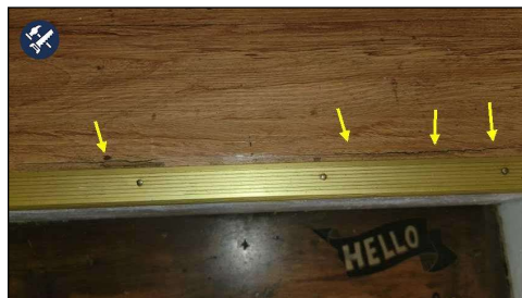
Cracking Observed.
