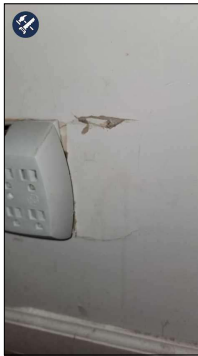
Dining Area--Damage to the Wall Observed(Cosmetic)
