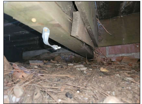
East Side--Almost Material to Soil
