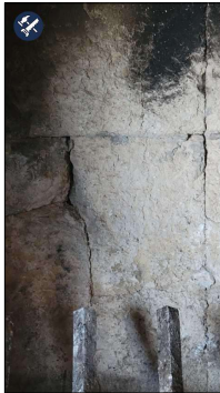
Dining Area--Damage to the Wall Observed(Cosmetic)
