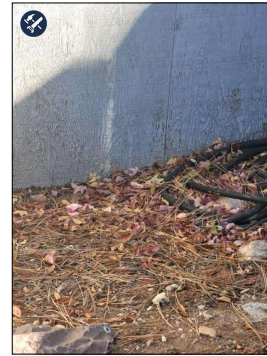
Siding is Material to Soil
