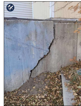
Retaining Wall is Cracked clean through and separating with a shift. On the the far west edge of th Property.
