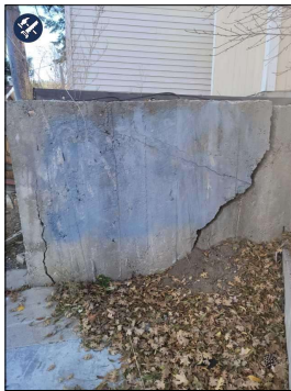
Retaining Wall is Cracked clean through and separating with a shift. On the the far west edge of th Property.
