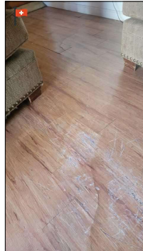
Living Room--Numerous Heavy Foundation Cracks Noted.
