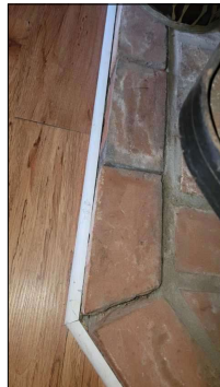
Bedroom#1--Cracks Observed in Brick Hearth.
