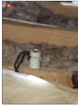
Old Knob & Tube in the Attic.
