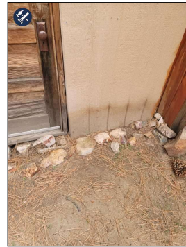
Shed Siding in the Rear of the Property
