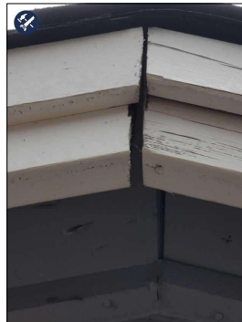
Fill & Seal All Gaps & Crack in the Eaves.
