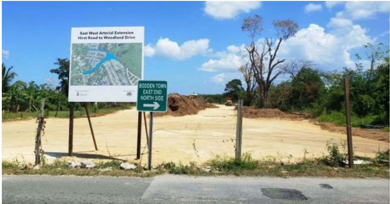
Figure 5. Construction of E-W Arterial Extension (Section 1)
