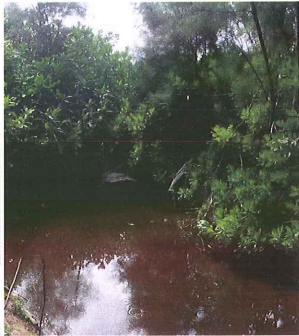
Fig 4: Landward End of South Sound Culvert
