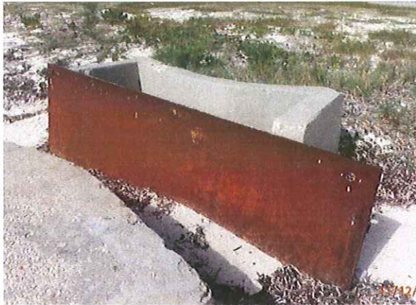
Fig 3: Closed Culvert in South Sound
