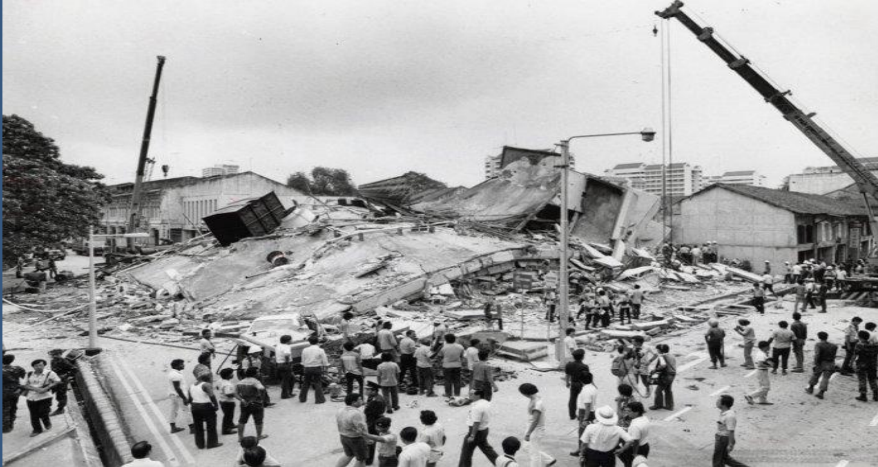
The collapse of the Hotel New World occurred on 15 March 1986, and was Singapore's deadliest civil disaster since the Spyros disaster on 12 October 1978
