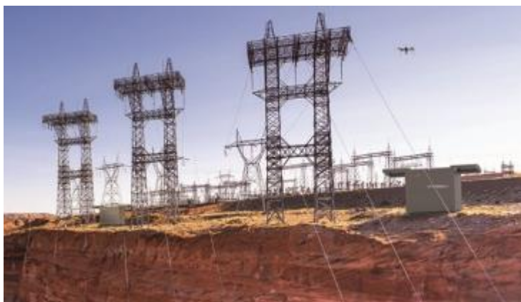
power grid inspection
