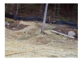
Stabilization of Steep Slopes with Erosion Control Blanket and Seed
