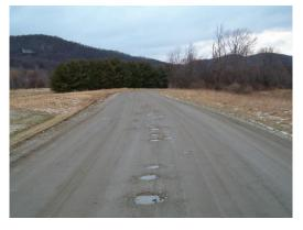
Views of Road Problems Created by Inadequate Stormwater Management Systems
