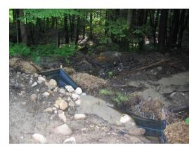
Sediment Overtopping the Silt Fence and Entering into Wetland
