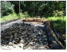
Trap Rock and Filter Fabric Placement through Wetland to Create an Unrestricted Flow
