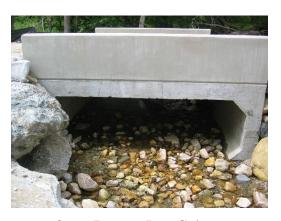
Open-Bottom Box Culvert for Stream Crossing
