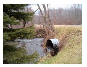
Views of Culvert Channeling Stream Flow Under Road
