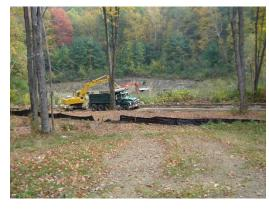
Loading De-Watered Sediments Into Dump Truck
