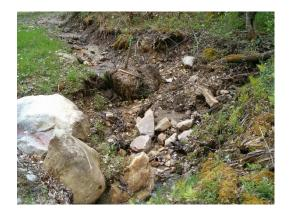
Washout along Common Drive due to Inadequate Swale Construction
