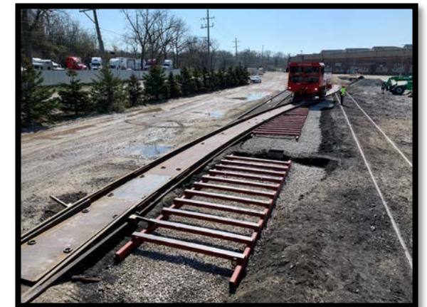
Open Rswitch, fine tune elevations
