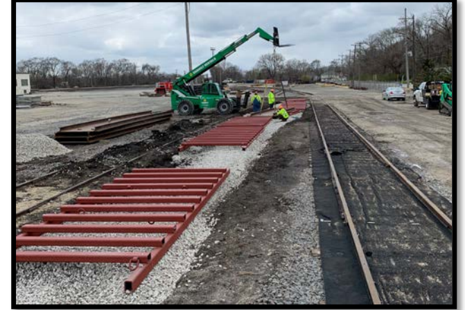
Grease top of Frames, Set Rswitch Panels, begin with pivot point and work outward
