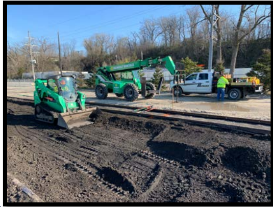
Excavate and Fill as Needed
