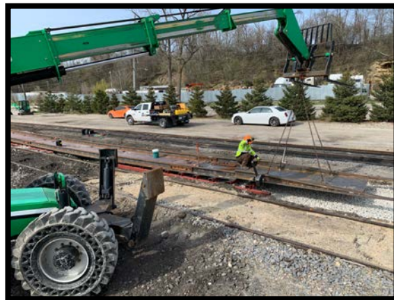
Bolt up Ramp Panels
