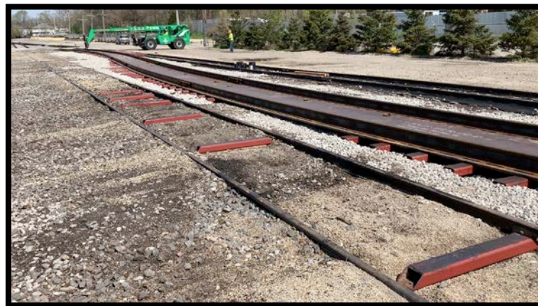
Lag bolt slide ties on top of main and siding ties
