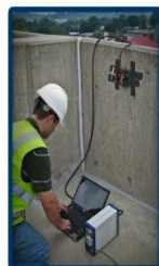
In-Situ Corrosion Rate Testing
