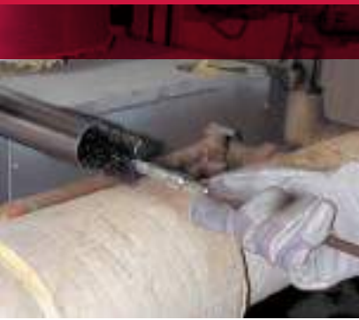
Cleaning boiler pipes with a flue brush.
