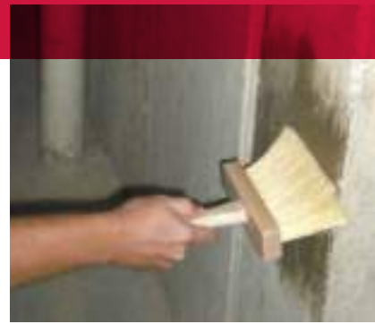
Applying waterproofing material with a masonry brush.
