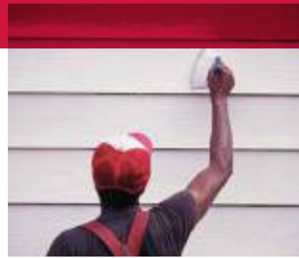
Applying paint to clap board siding.
