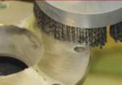
Removing gasket material from a pipe flange.
