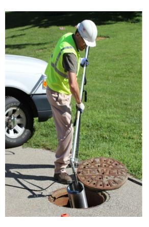
Installation of a Micro-Meter
