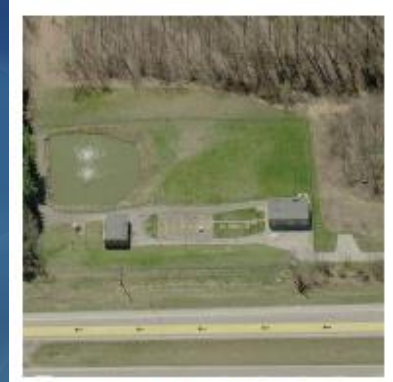
AUBURN CORNERS WWTP
