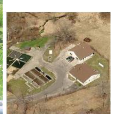
INFIRMARY CREEK WWTP
