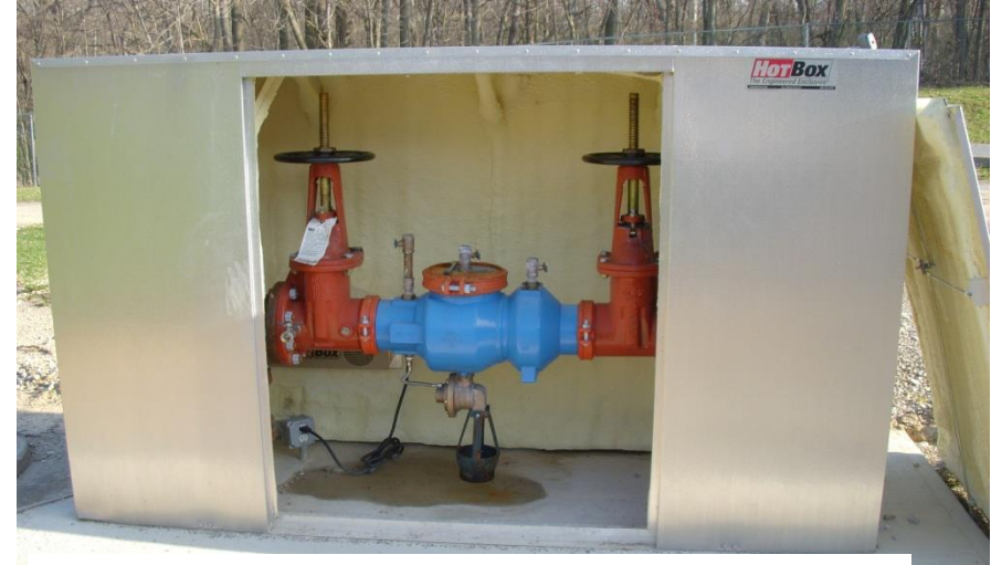
Reduced Pressure/Detector Assembly
