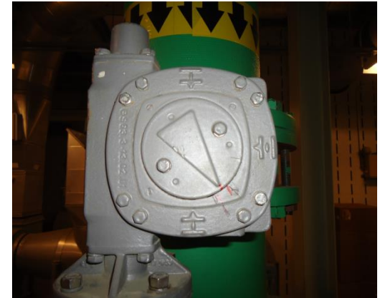
Inlet valve throttled 30%
