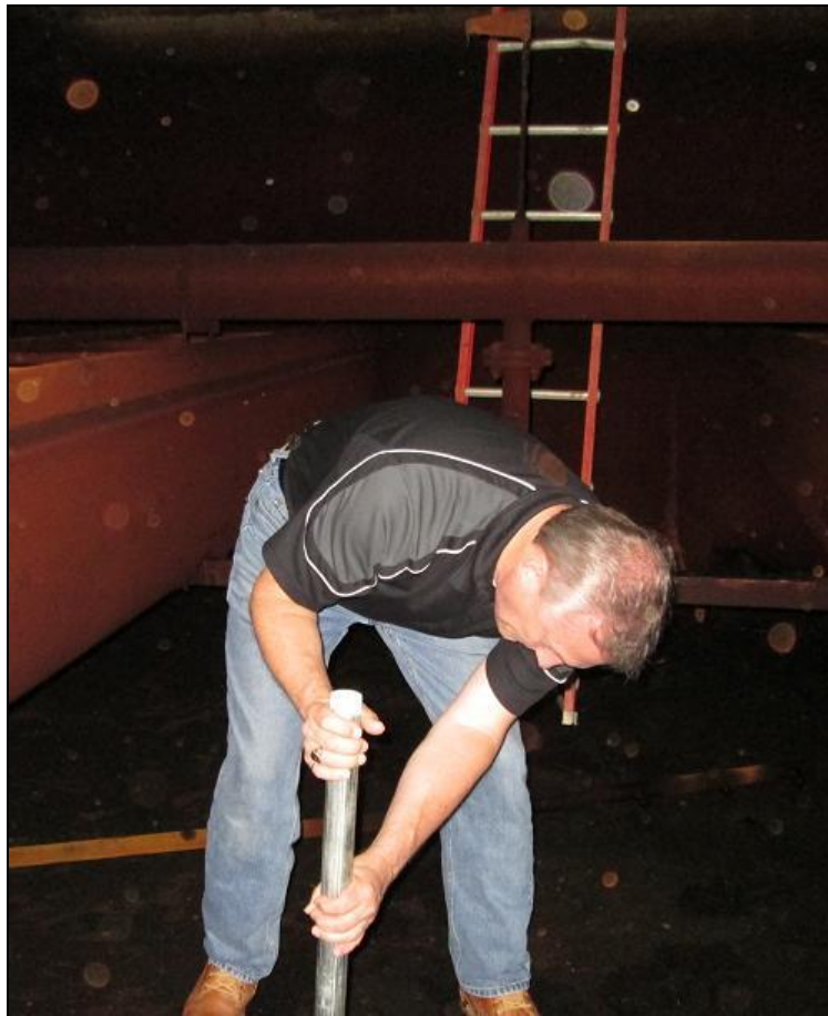
Media coring in filter bed
