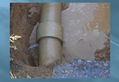
Leaking collars on asbestos cement pipe
