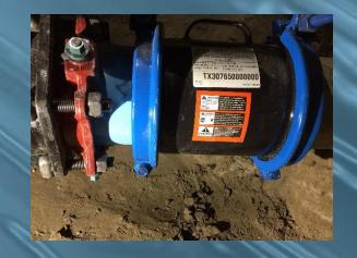
Deflection: Up to 4 degrees per end 3/8" longitudinal movement allowed (equivalent to a 120 degrees temperature rise on steel pipe)
