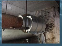
Completed Encapsulation and Insulation of Flange to Prevent Freezing
