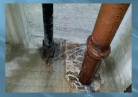
Lead Calk Bell on Old Cast Iron Pipe
