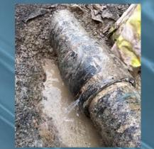
Ductile Iron Push-On Joint
