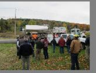
Engineers and operators from all over New England and upstate New York were invited to observe the work and learn about the new and innovative pigging process.
