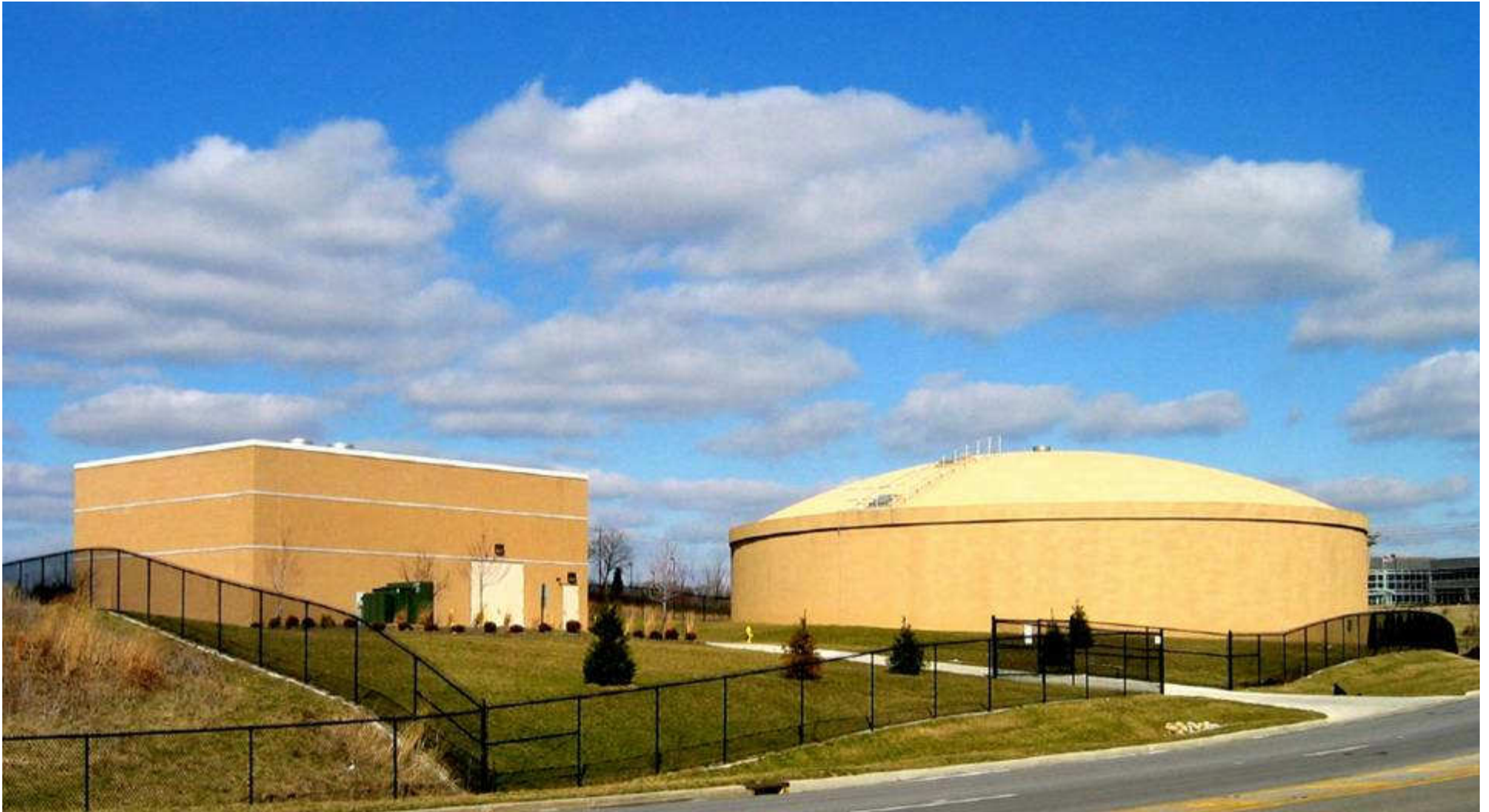
Mason, OH Water Storage Tank 2003 2.0 MG 122' diameter x 23' swd Owner: Greater Cincinnati Water Works Engr: Gannett Fleming
