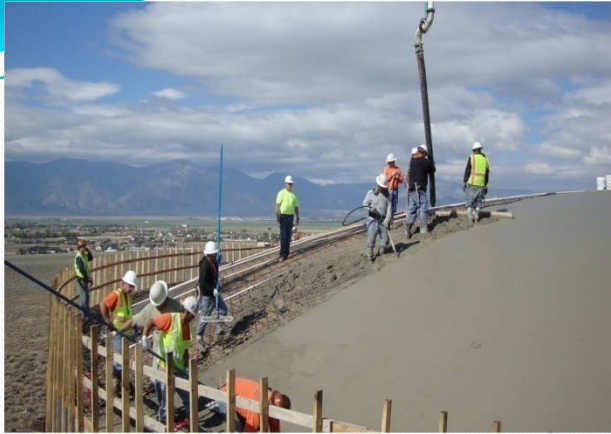
Cast In Place
