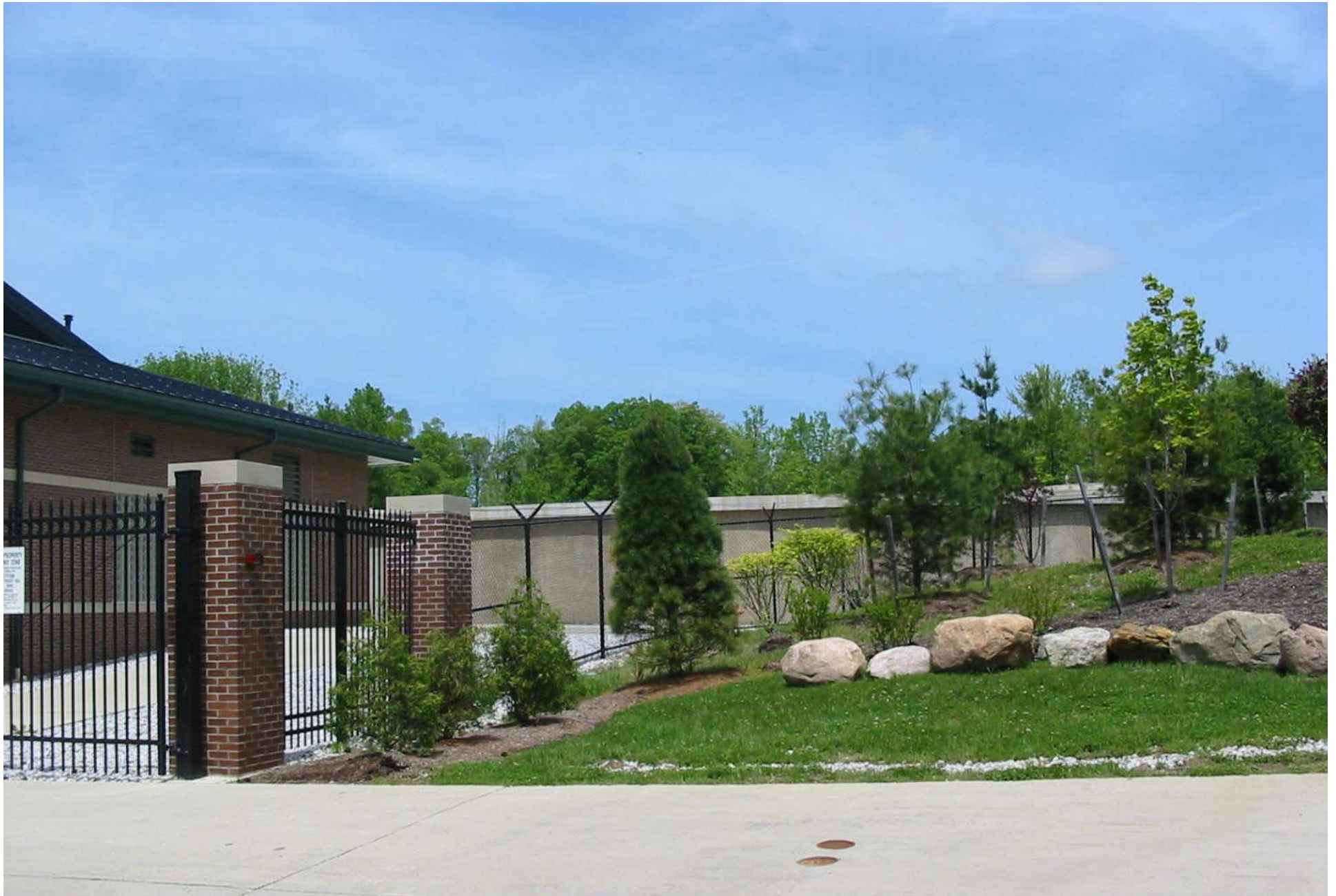
North Royalton, OH 2000 Owner: Cleveland Div of Water 5.0 mg WST (2.0 / 3.0) 212' diam x 20' swd Engr: AECOM (M & E)
