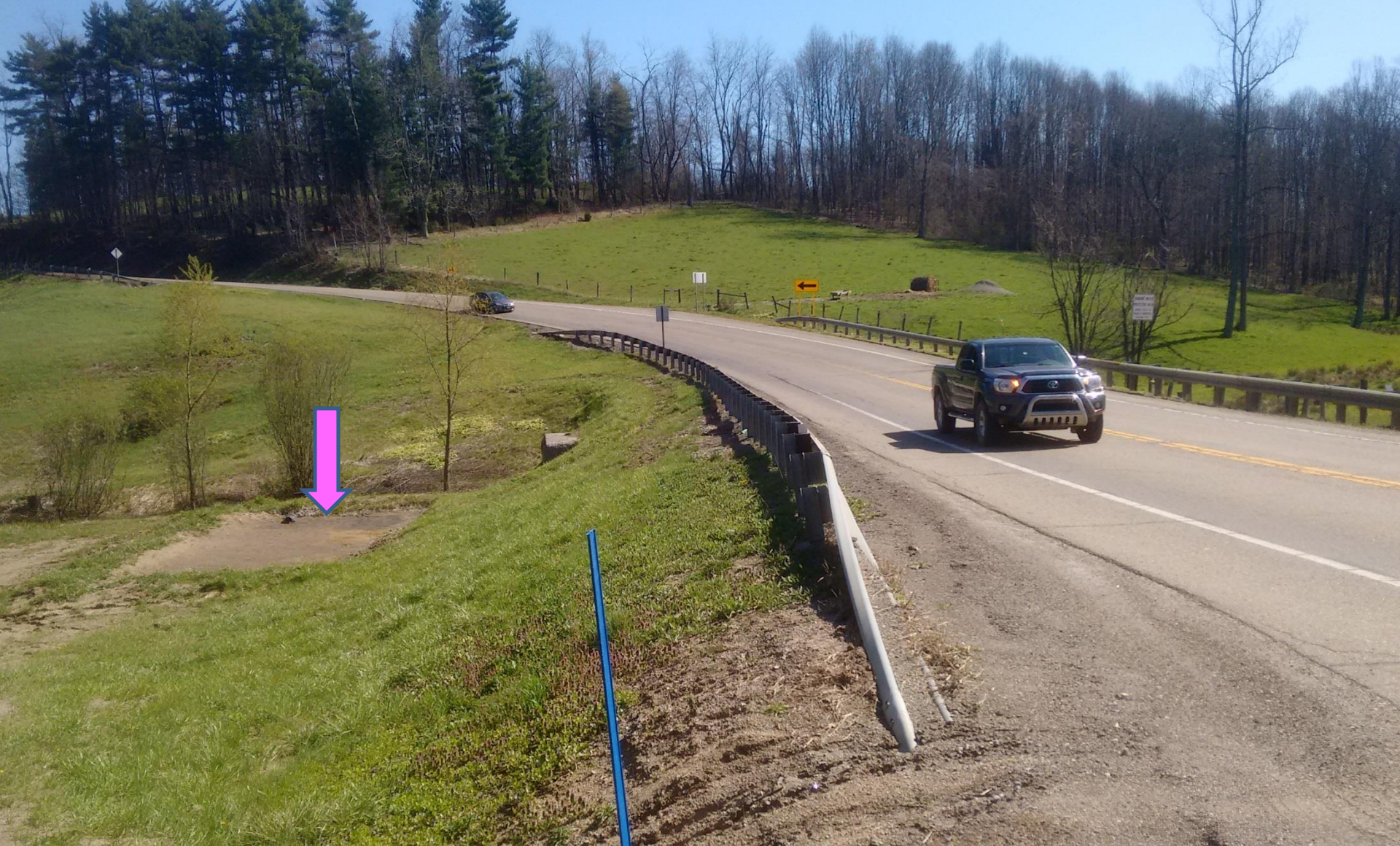
Barnesville, 2016 Spill Impoundment, east side of SR 800
