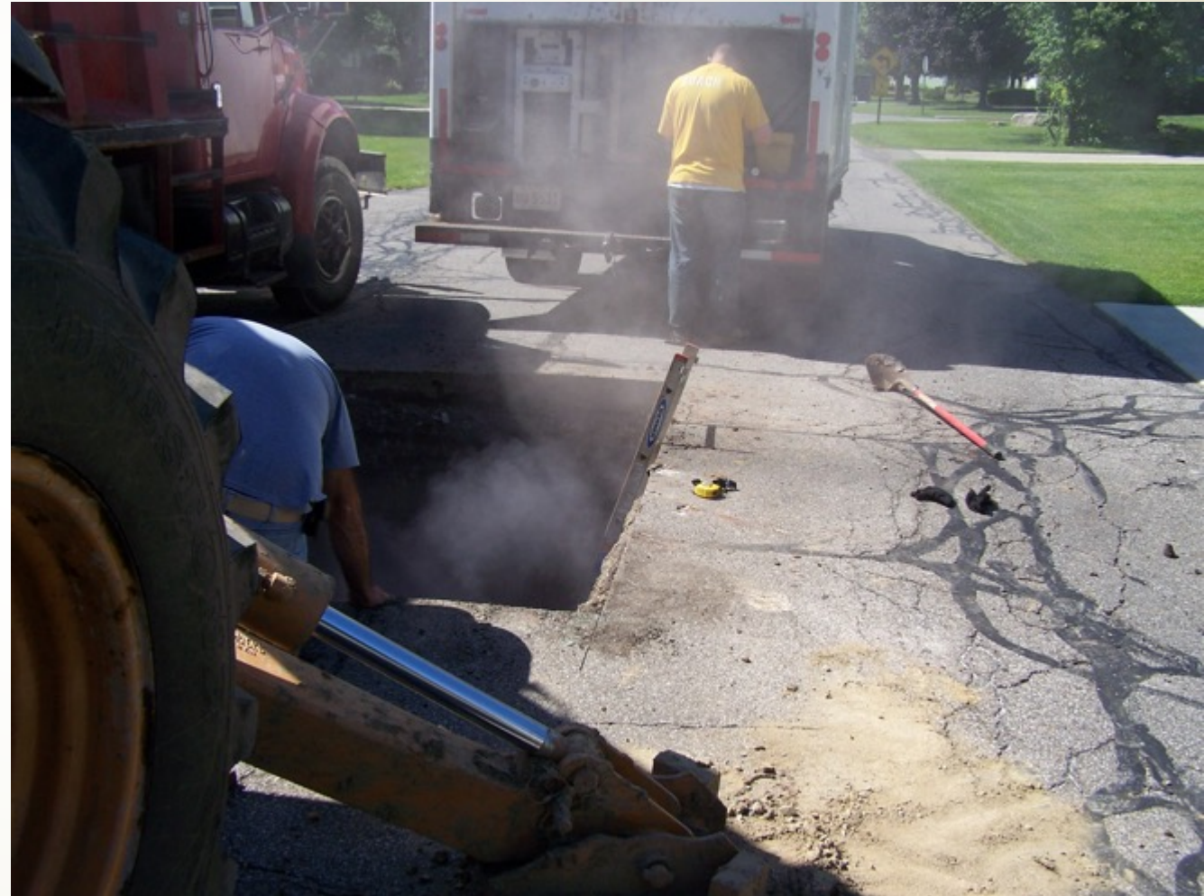
Trenching to access a sewer line is through previously disturbed soil.
