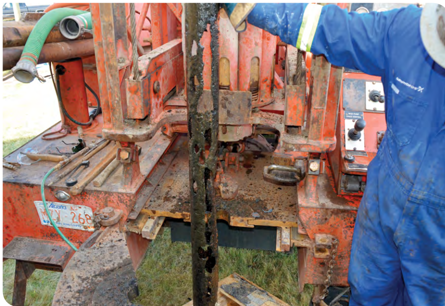
Figure 7-2, Holes in Well Casing
