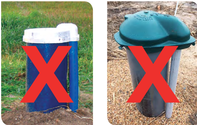
Figure 4-5, Examples of Standard Well Caps
