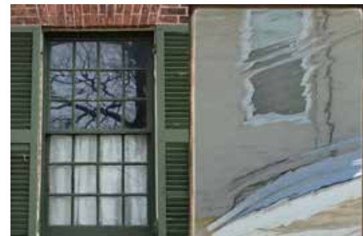
Twelve over 12 window (left) with close up of crown glass pane (right). (Supplied photo)
