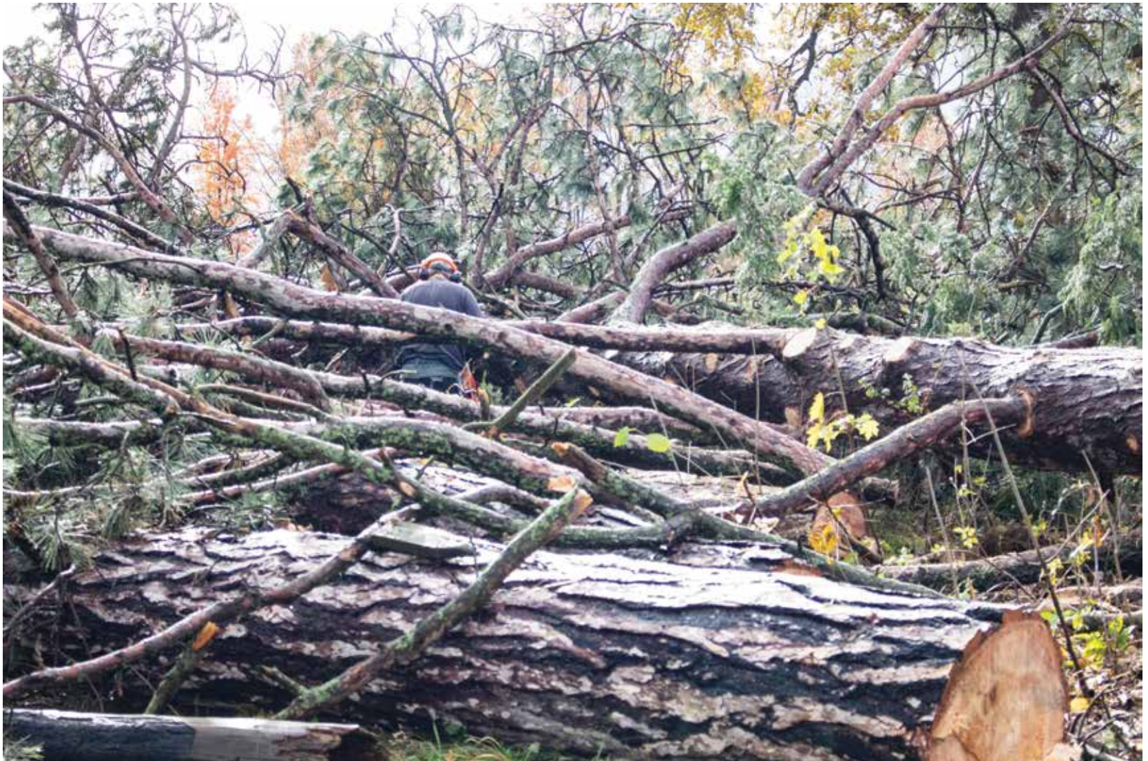
A tree service worker saws through healthy trees at 200 John St. behind the Randwood Estate, on a property expected to be the future location of a subdivision by Solmar Development Corp. (Richard Harley)
