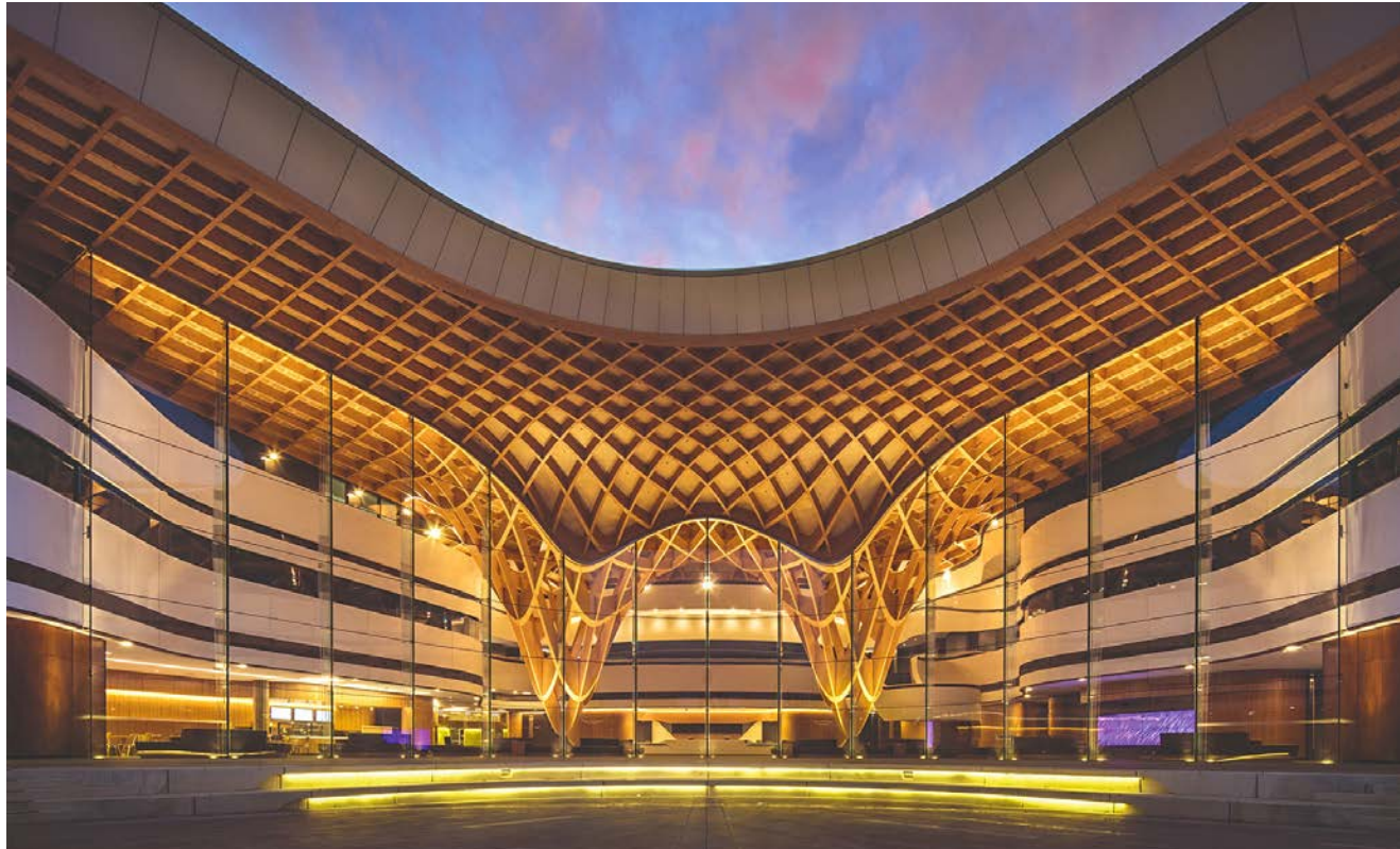
Architectural artistry expressed through the medium of massive timber. BLUMER LEHMANN AG
