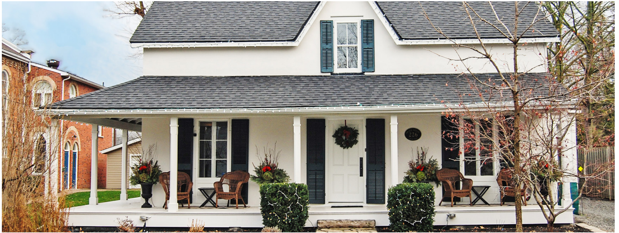
This Ontario Gothic Cottage at 226 Victoria St. shows the typical form and verandah. Brian Marshall says it's a great example of the architectural style. SUPPLIED
