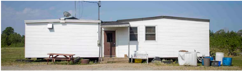
The bunkhouse on Read Road where a farmworker died last week. SOMER SLOBODIAN
