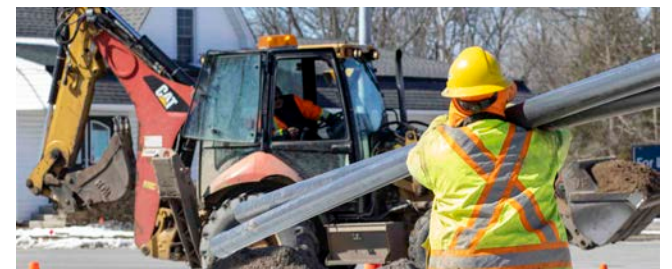
Construction is backing up traffic in Virgil. SOMER SLOBODIAN
